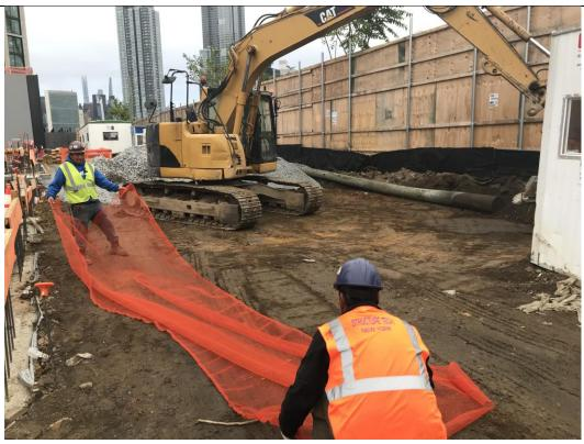
View of STNY backfilling with 0.75-inch and 2.5-inch virgin stone in waste characterization COMP K (facing north)
