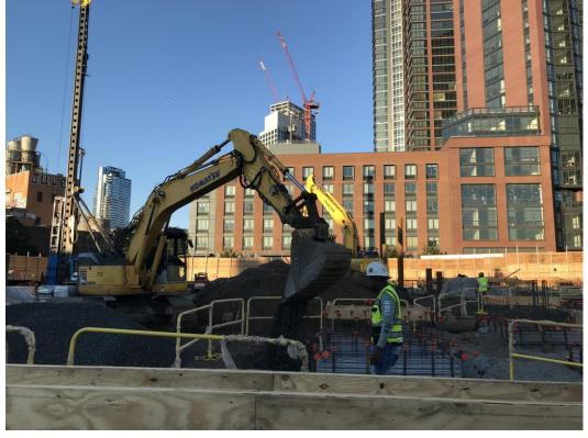
View of STNY installing Grace Preprufe® 300R waterproofing/vapor barrier waterproofing the mat slab (facing south).
