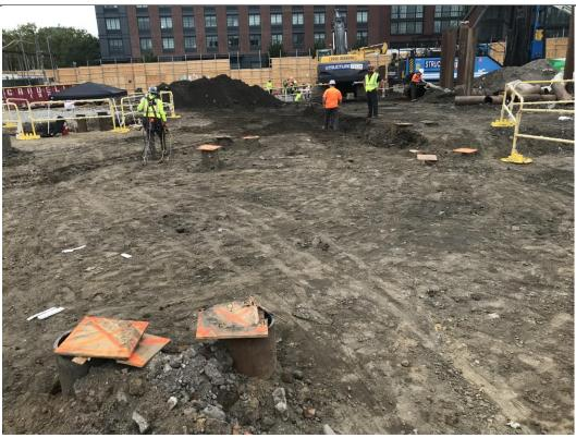
View of STNY excavating to install pile cap formwork in waste characterization grid COMP G (0-5) (facing north).
