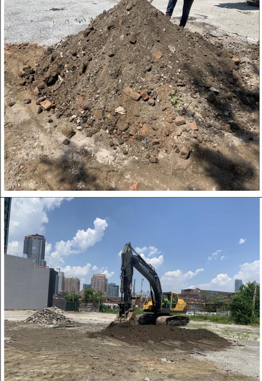
**Photo 4:** View of STNY backfilling the test pit excavation at the LB22 hotspot, located in the central part of the site (facing northeast).
