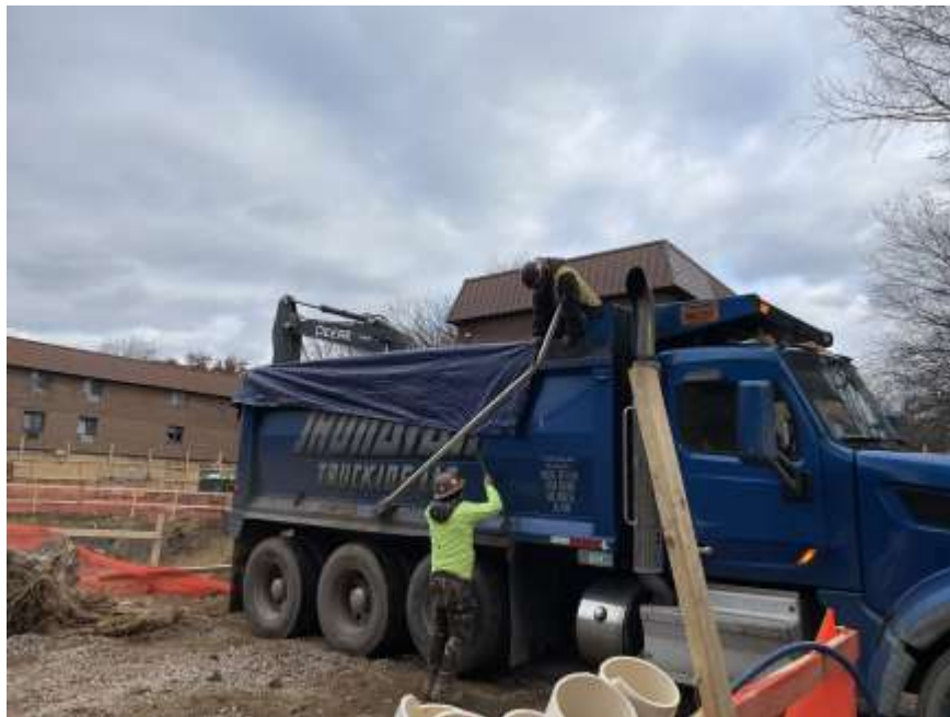
Photo 2: View of permitted tri-axle truck transporting non-hazardous fill for off-site disposal. Trucks were securely covered and tires washed prior to leaving the site (facing northeast).
