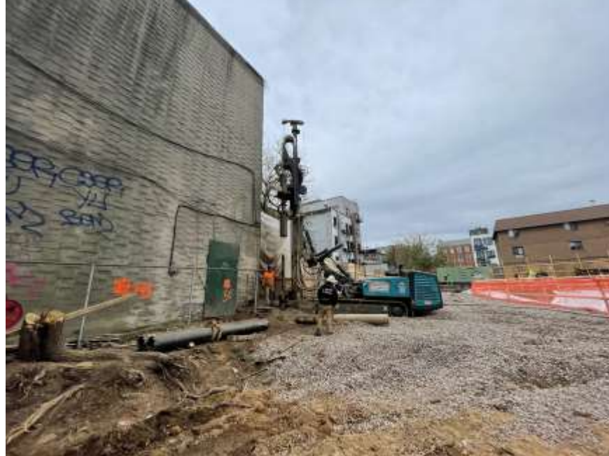
Photo 1: Anel installing soldier piles along the western site boundary (facing north).
