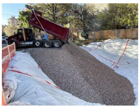
**Photo 1:** View of Rise importing 34-inch RCA imported for construction of the temporary equipment ramp in the central part of the site (facing southwest).
