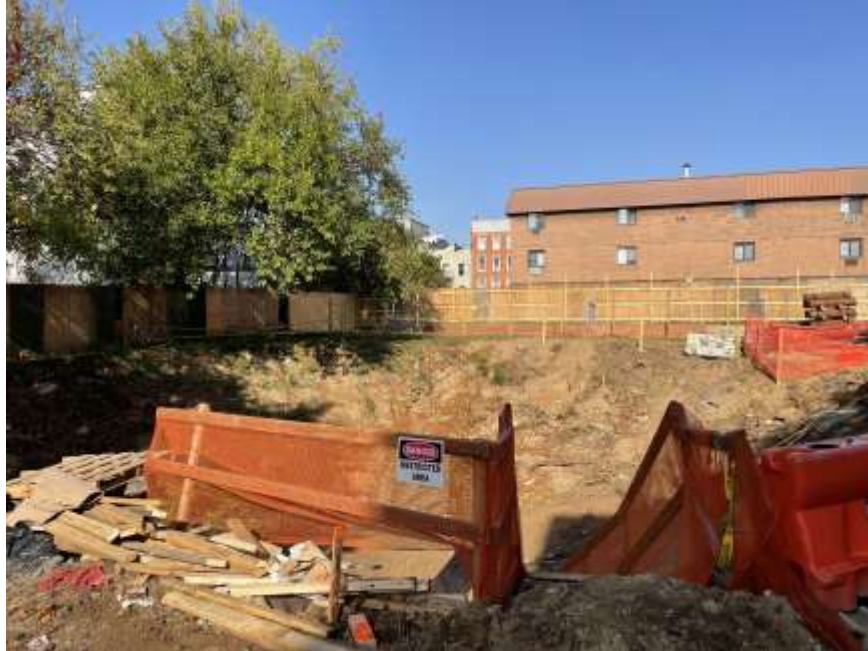
Photo 1: General view of the site (facing north).
