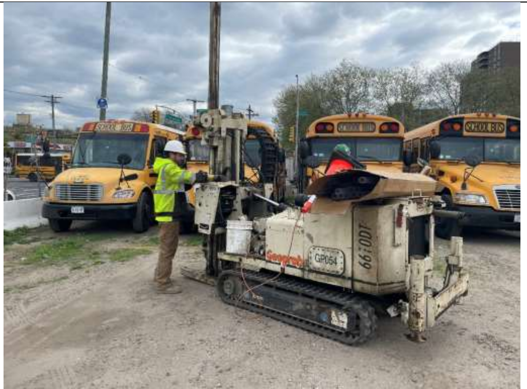
Photo 1 – AARCO drilling LSB-20A, facing northeast.
