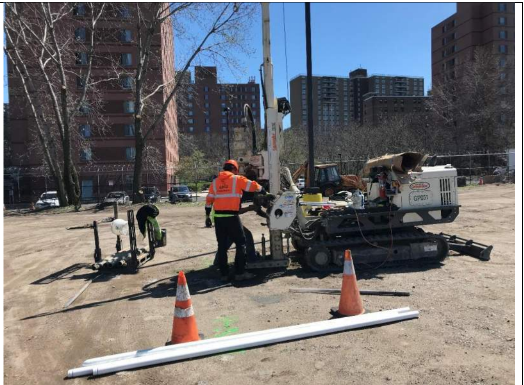
Photo 3 – Drilling soil boring LSB-25, facing southeast.
