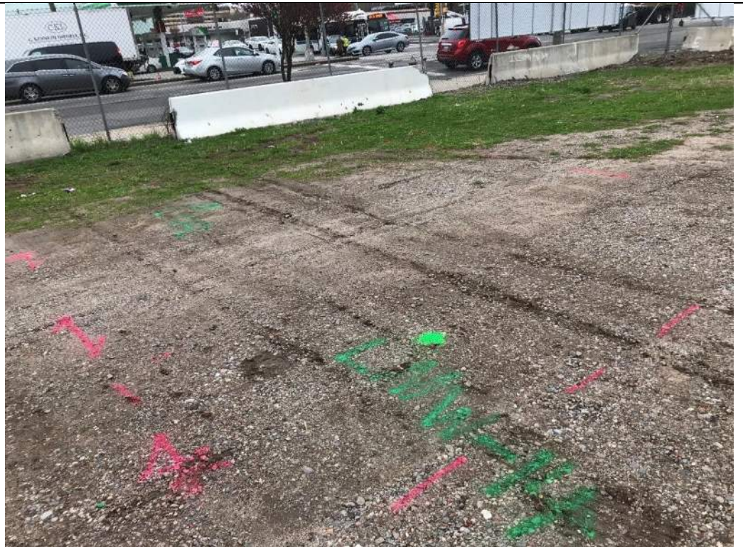
Photo 4 – Utility mark-out within the vicinity of proposed LMW-14/LSV-2 locations.
