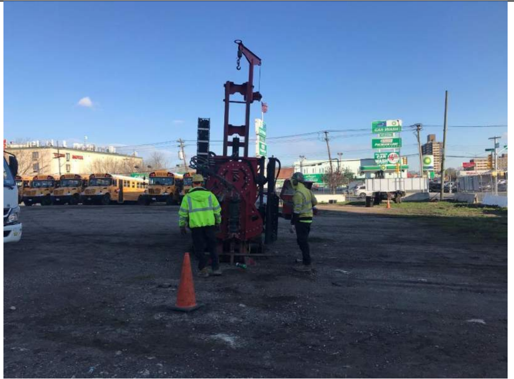
Photo 1 – Drilling for installation of soil vapor point LSV-5, facing northwest.
