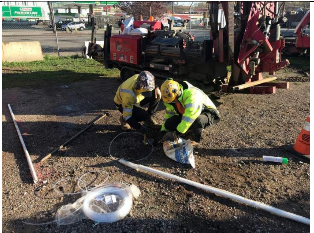
Photo 2 – Installation of soil vapor monitoring point at LSV-2, facing north.
