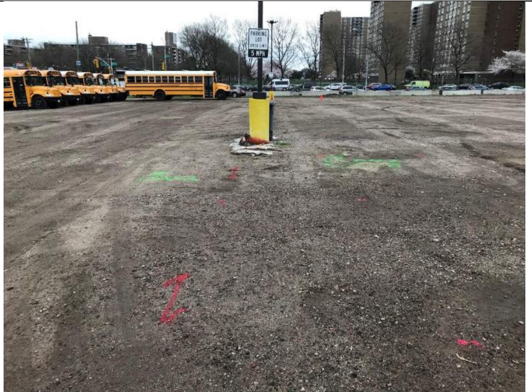
Photo 3 – Utility mark-out within the vicinity of proposed LSB-22/LMW-8/LSV-3 locations.
