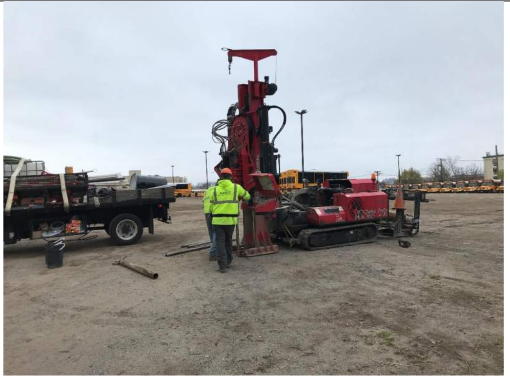
Photo 1 – Drilling soil boring LSB-24, facing west.
