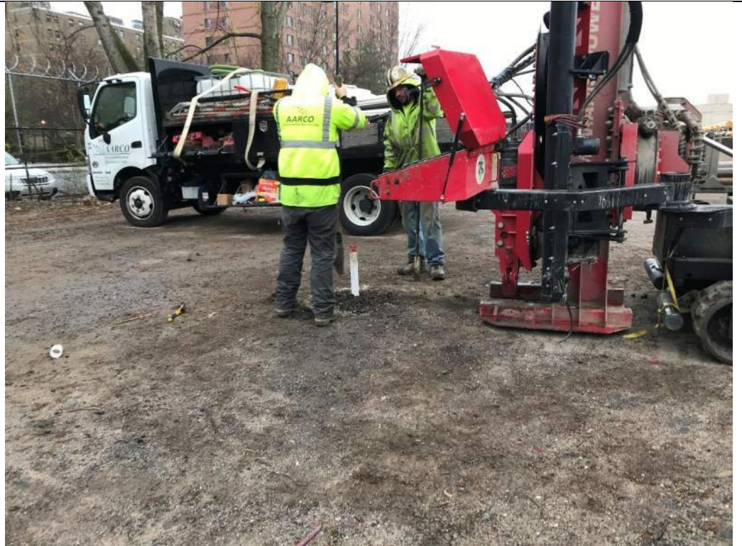
Photo 3 – Installing LMW-13, facing south.
