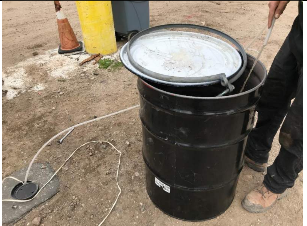
Photo 3 – Developing monitoring well LMW-8, facing west.
