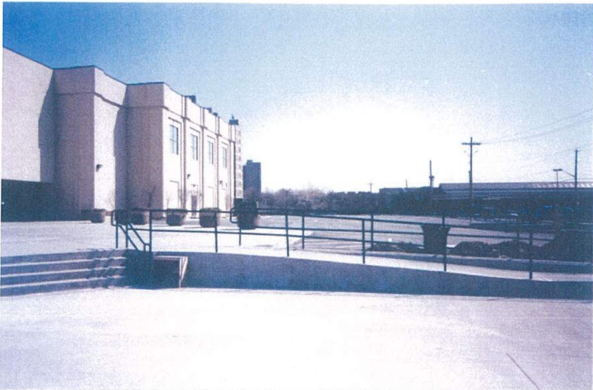
VIEW OF WEST SIDE OF BUILDING AND PARKING AREAS
