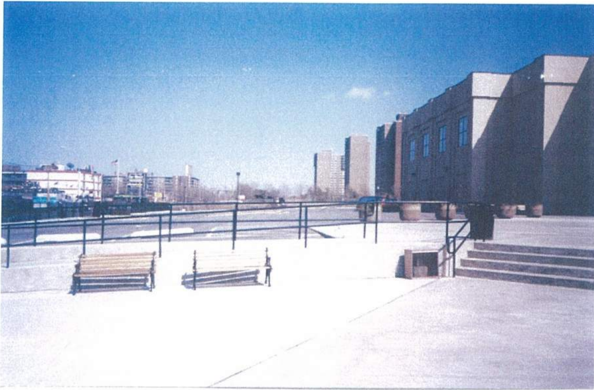
VIEW OF NORTH SIDE OF BUILDING AND PARKING AREAS
