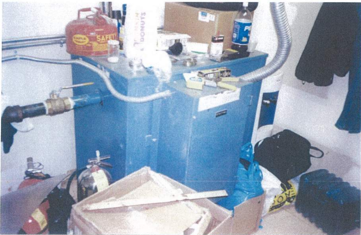
VIEW OF ELEVATOR MOTOR UNIT
