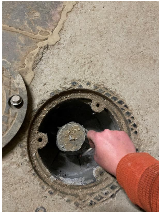
Photo 10, 11/29/2023: View of smoke testing (facing down).
