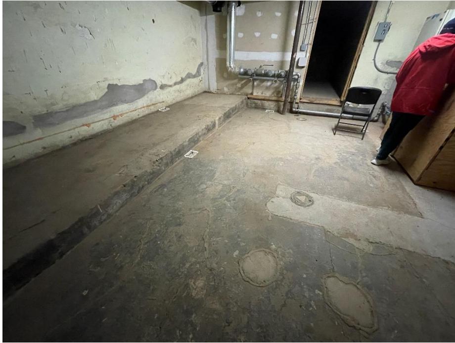
Photo 9, 11/29/2023: View of cellar (facing west).
