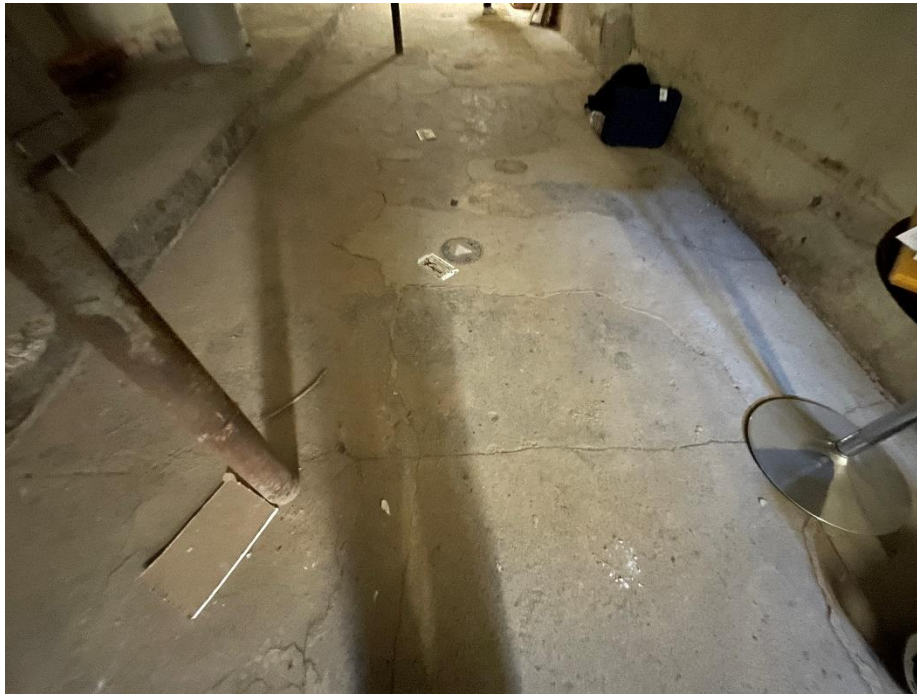
Photo 1, 11/29/2023: View of cellar (facing west).
