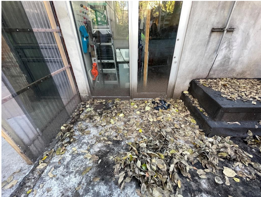
Photo 5, 11/29/2023: Rear-yard composite cover (facing east).
