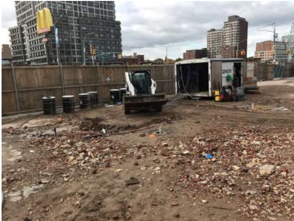
Photo 1: Bobcat clearing demo debris to uncover monitoring well MW-112, looking southwest.
