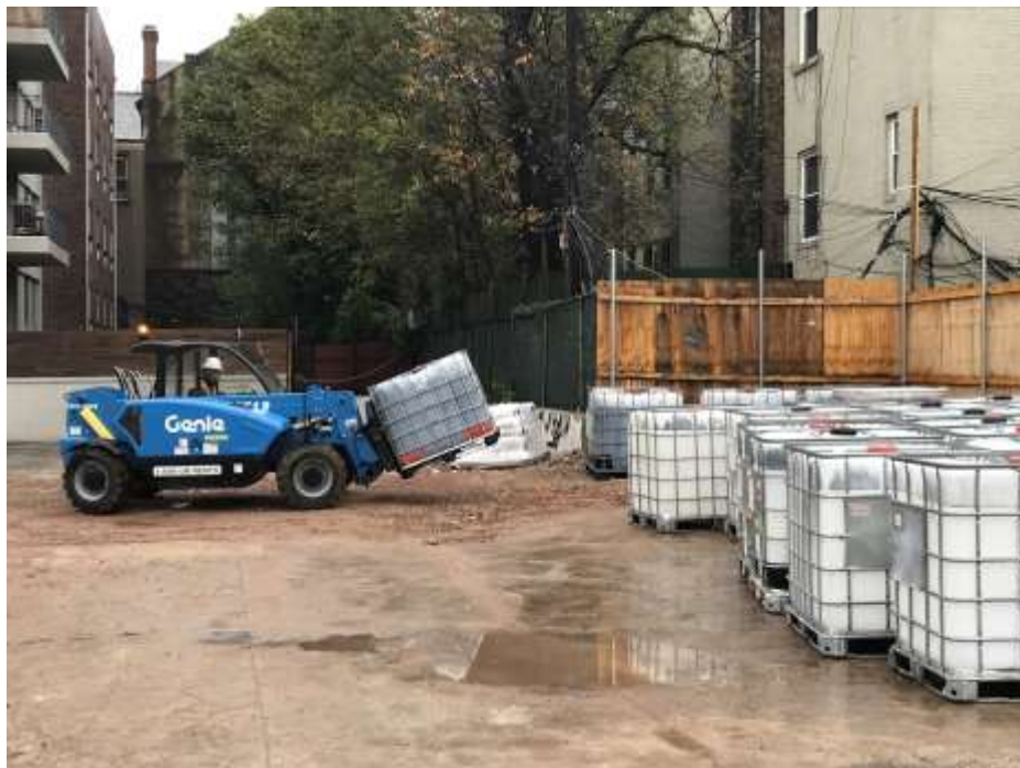
Photo 2: Regensis using a forklift to move PlumeStop totes to the injection area.
