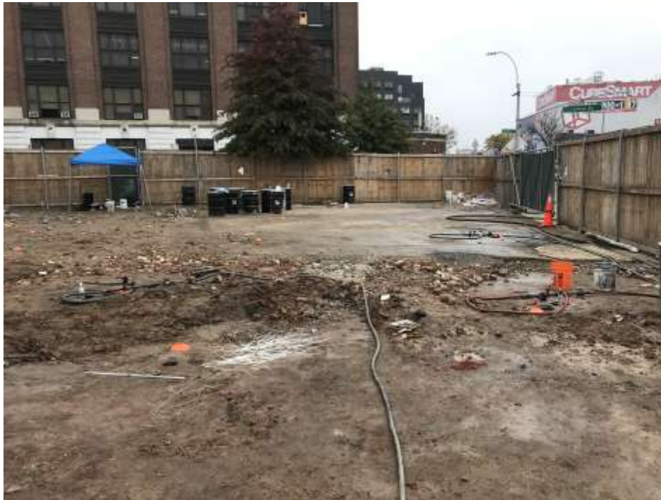
Photo 1: Hoses connected to injection points IP-01, IP-03, IP-04, and IP-09, looking east.
