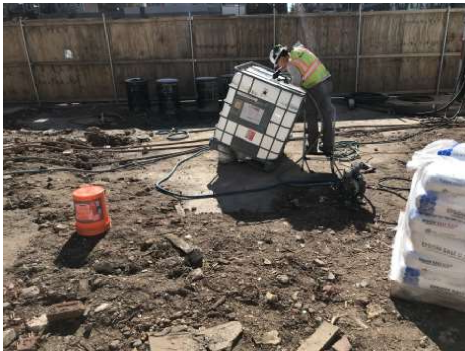
Photo 2: Regeneration mixing and injecting Nutrisulfate at IP-04, looking south.
