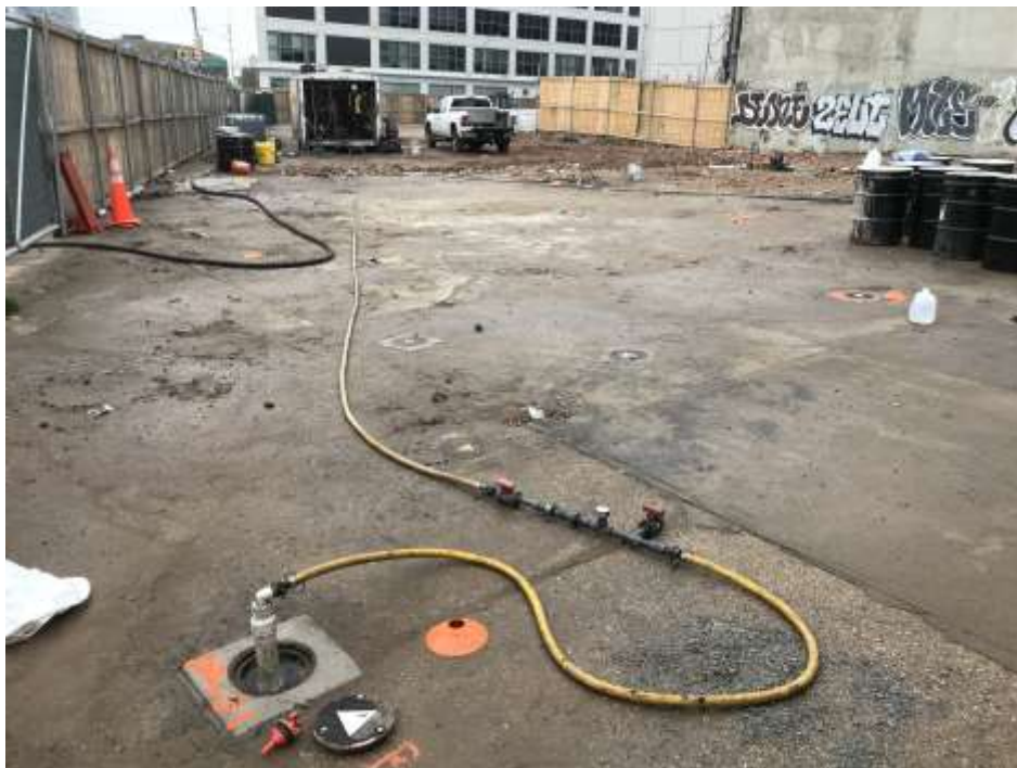
Photo 2: Hose connected to injection point IP-01, looking west.
