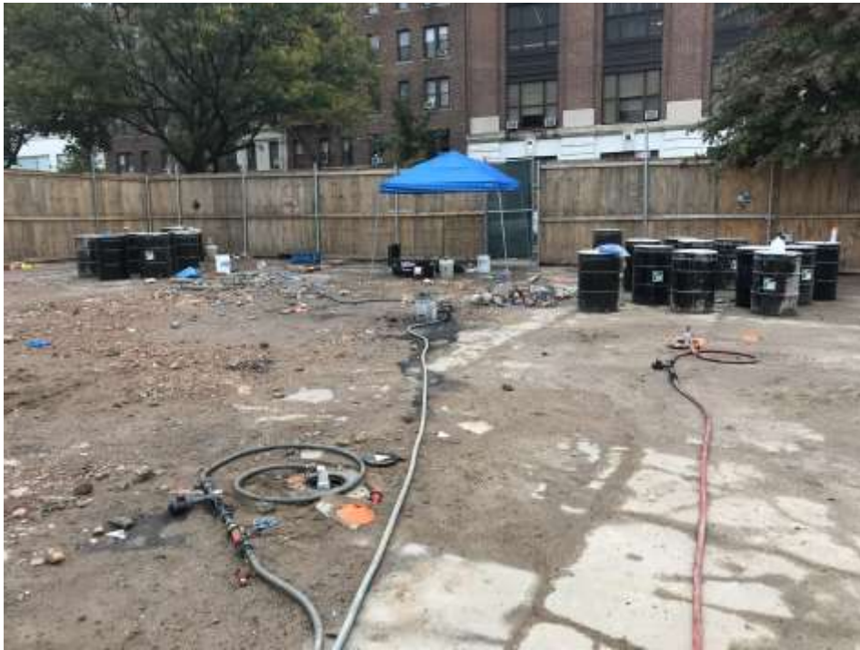
Photo 1: Hoses connected to injection points IP-07, IP-08, and IP-12, looking northeast.
