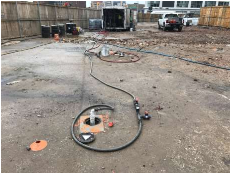
Photo 1: Hoses connected to injection points IP-07 and IP-08, looking west.
