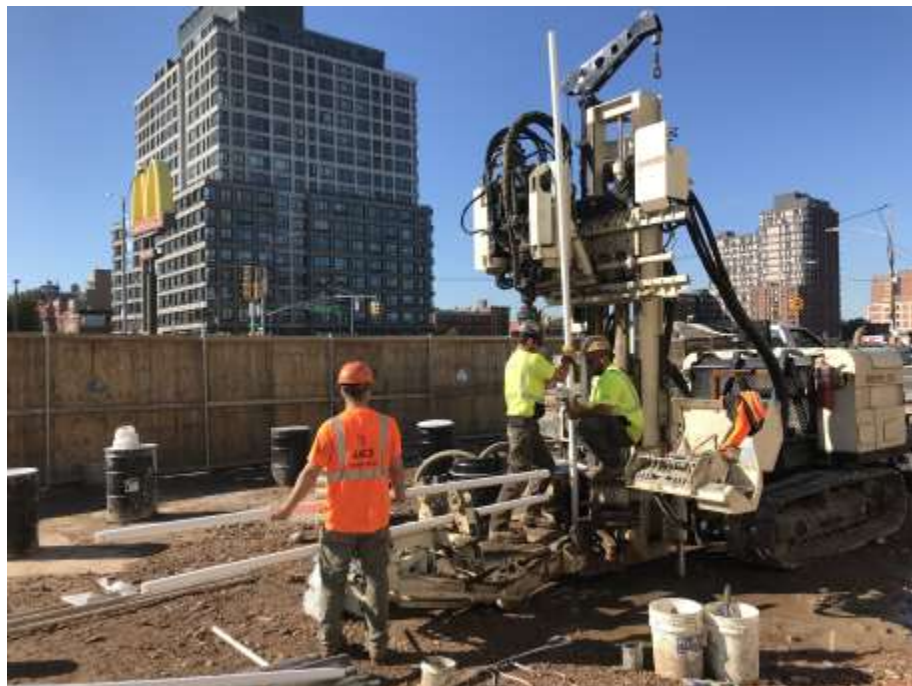
Photo 1: AARCO installing well IP-10 (facing southwest).
