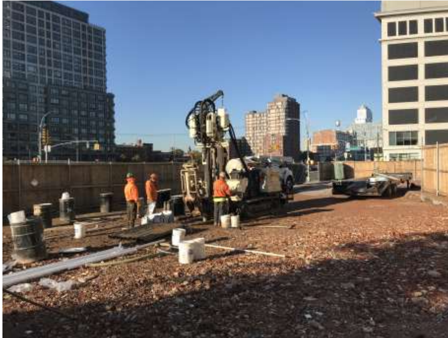
Photo 2: AARCO advancing boring IP-10 (facing west).
