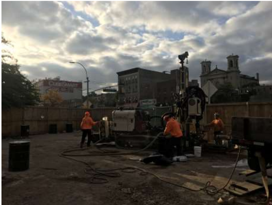
Photo 1: AARCO advancing boring IP-03 (facing southeast).
