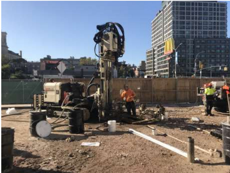
Photo 1: AARCO advancing boring IP-08 (facing south).
