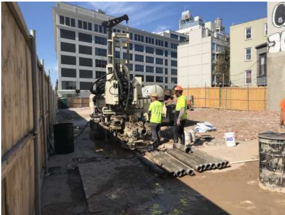
Photo 2: AARCO advancing boring IP-04 (facing west).
