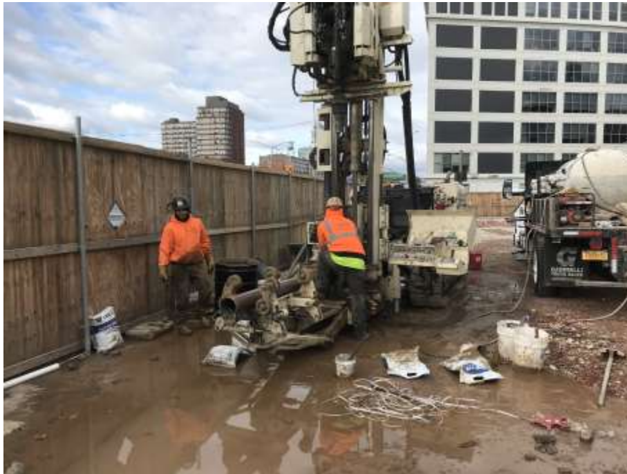
Photo 1: AARCO installing injection well IP-05 (facing west).
