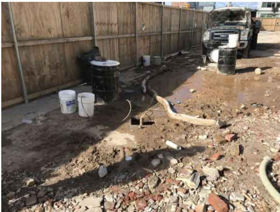
Photo 2: AARCO developing injection well IP-08 (facing west).
