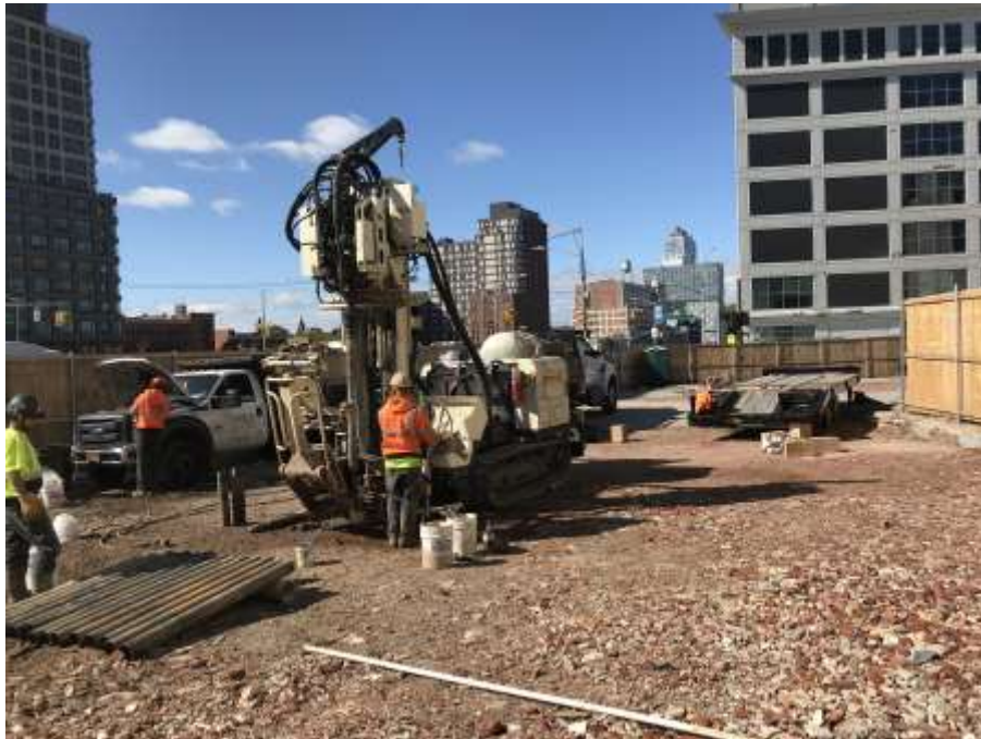
Photo 1: AARCO advancing boring IP-10 (facing west).
