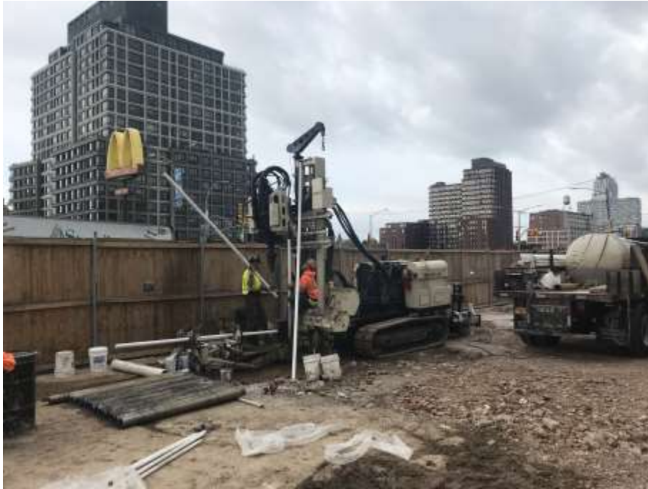
Photo 1: AARCO installing injection well IP-04 (facing southeast).
