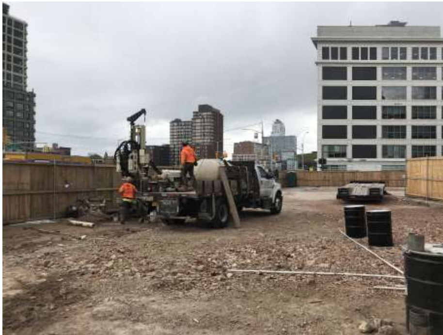
Photo 2: AARCO advancing boring IP-05 (facing west).
