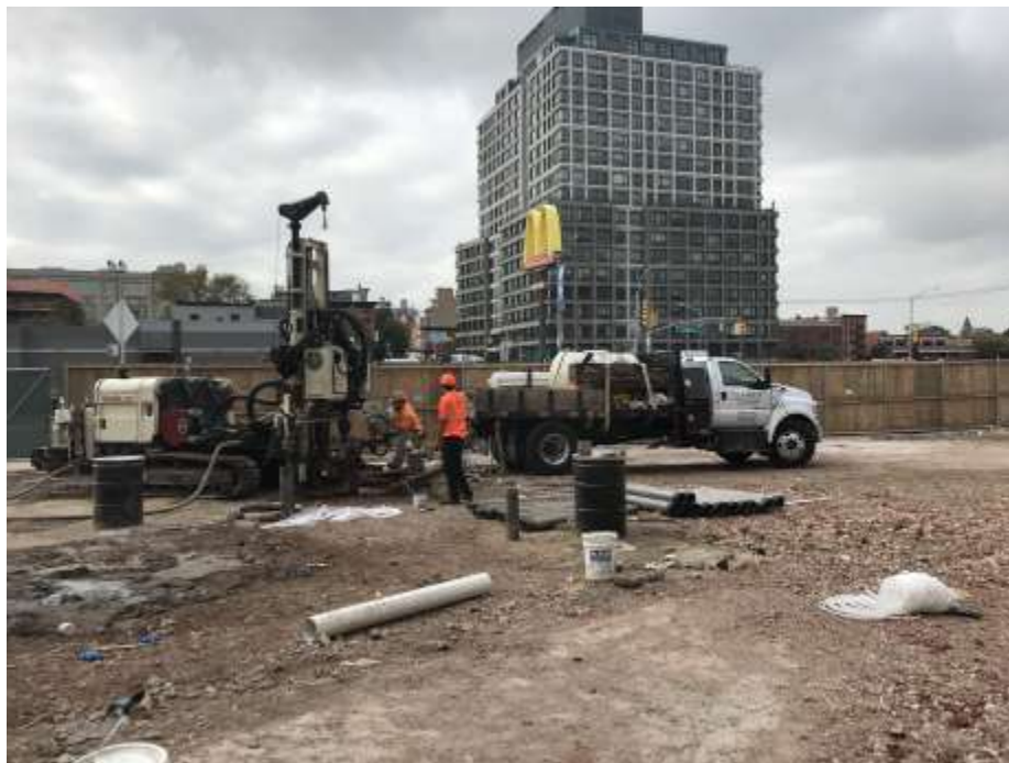
Photo 2: AARCO advancing boring IP-08 (facing south).
