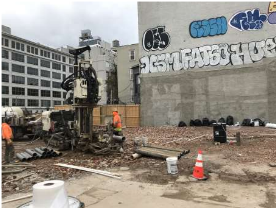
Photo 2: AARCO advancing boring IP-09 (facing northwest).
