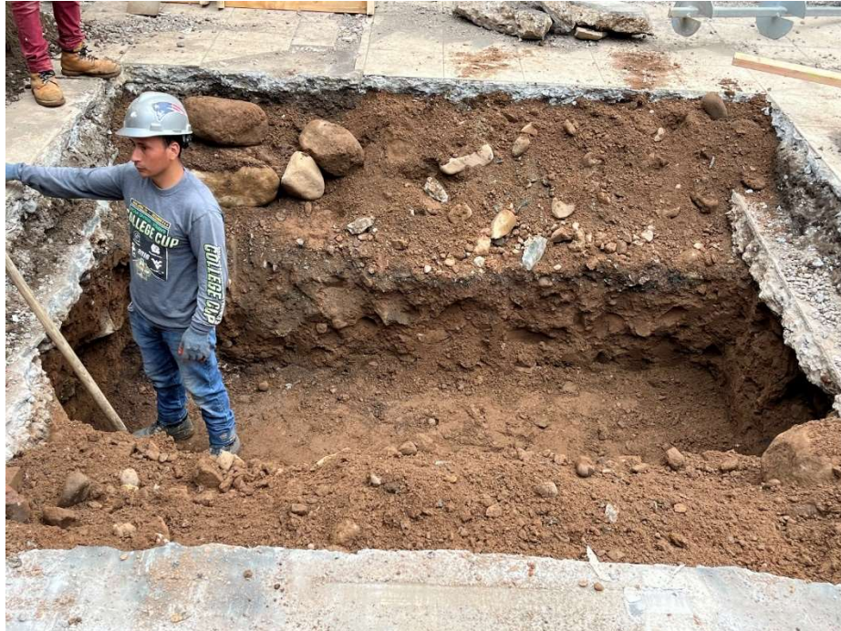
Photo 2: View of the completed excavation for pile installation (facing north).
