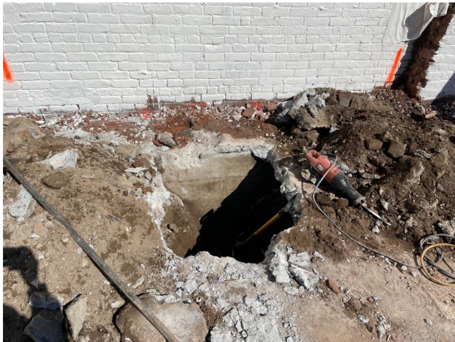
Photo 2: View of a representative test pit (facing north).
