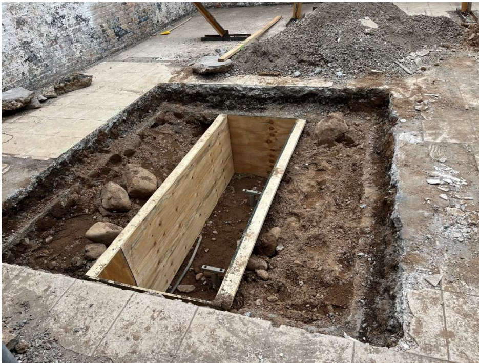
Photo 4: View of formwork and installed piles in excavation (facing northeast).
