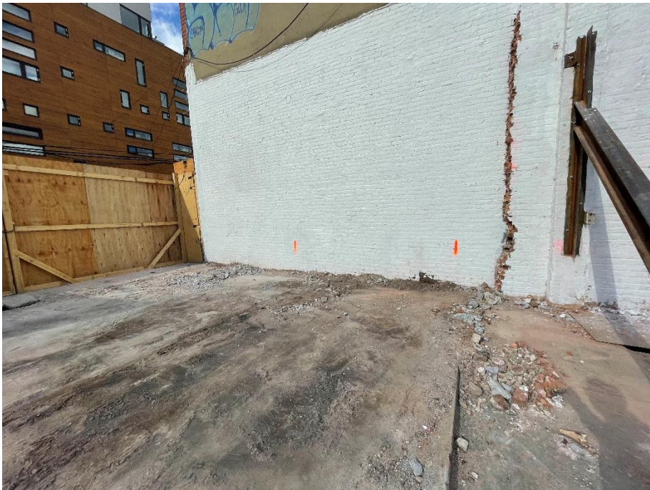
Photo 2: View of the backfilled test pits (facing northwest).
