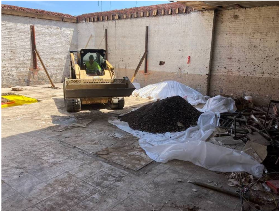
Photo 1: View of RYBAK stockpiling gravel subbase (facing northeast).
