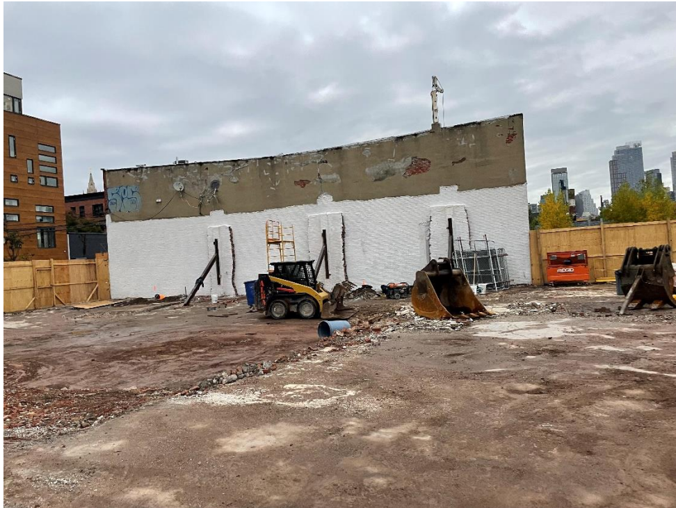
Photo 1: General view of the site (facing northwest).
