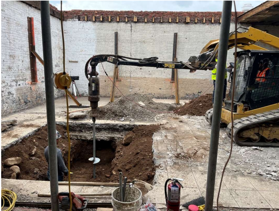
Photo 3: View of RYBAK installing helical piles into excavation (facing east).
