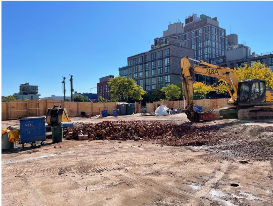
Photo 1: General view of the site (facing southeast).
