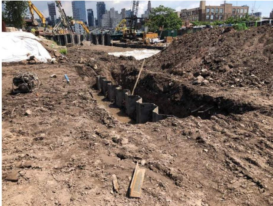
Photo 2: View of trench excavated for the installation of deadman wale no. 6 (facing northeast).
