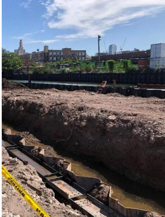
Photo 3: View of the sheet pile deadman and wale installation progress (facing northeast).
