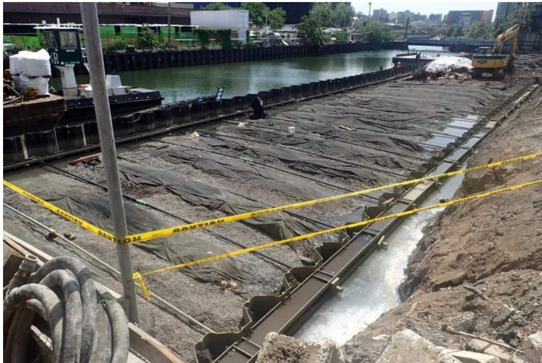
Photo 1: View of tie rods with corrosion protection tape applied (facing east).
