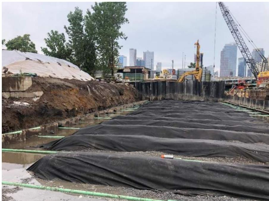
Photo 2: View of the tie rod installation progress in the northern region of the site (facing northeast).
