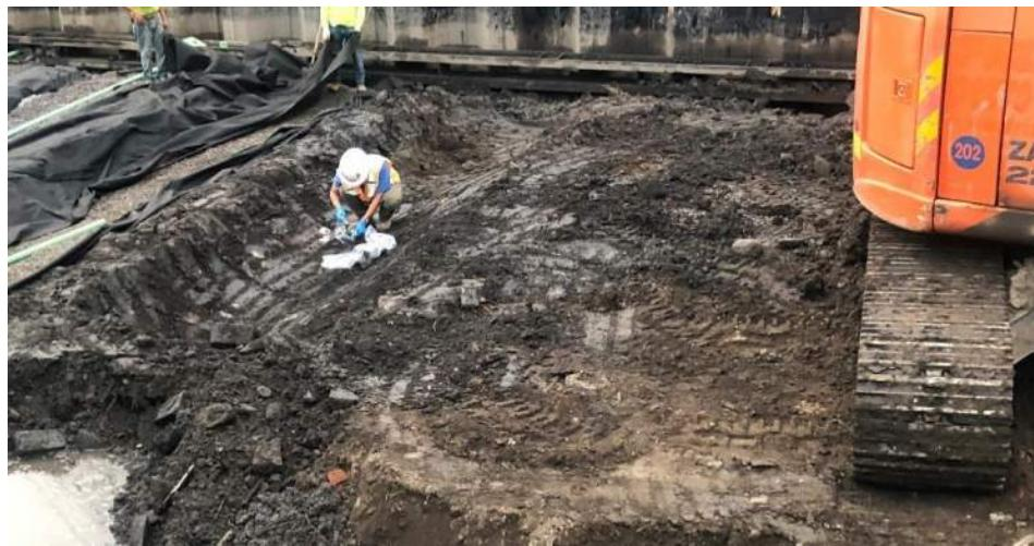
Photo 1: View of Langan collecting soil samples from the base of the tie rod trench excavation (facing east).
