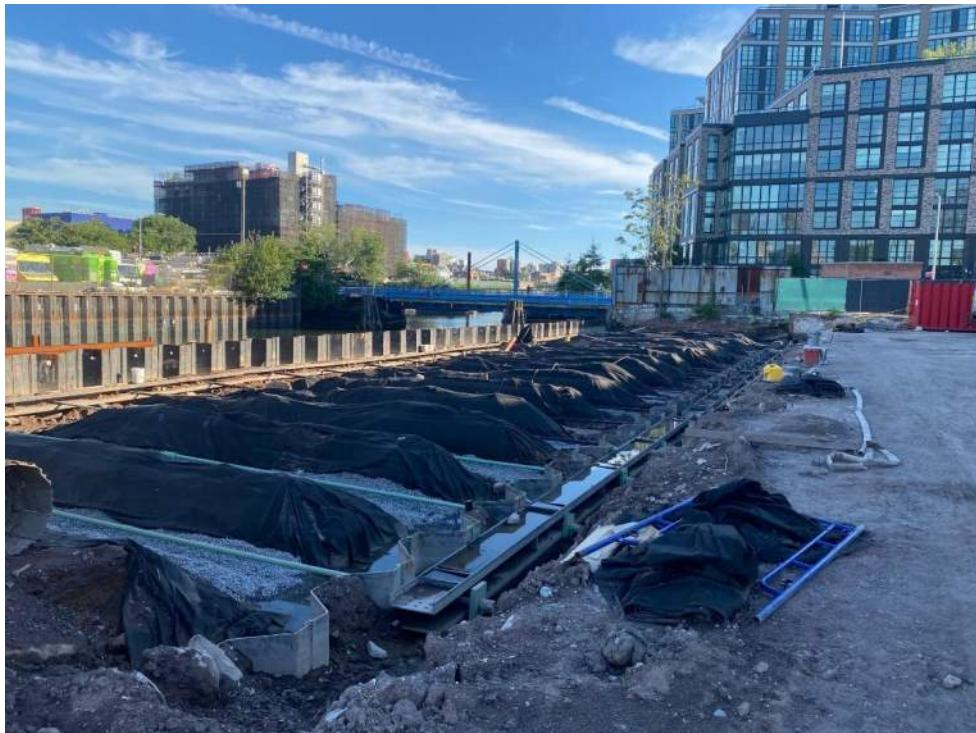
Photo 1: View of tie rod installation progress along the southeast region of the site (facing southeast).
