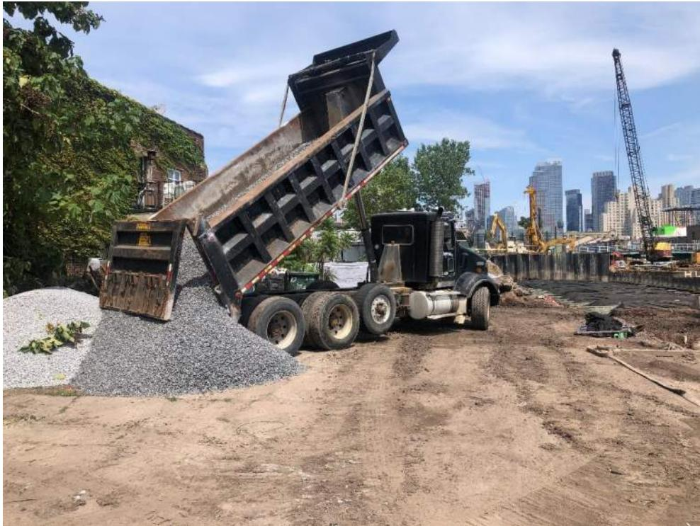
Photo 2: View of ¾-inch virgin quarry stone being imported to site (facing northeast).
