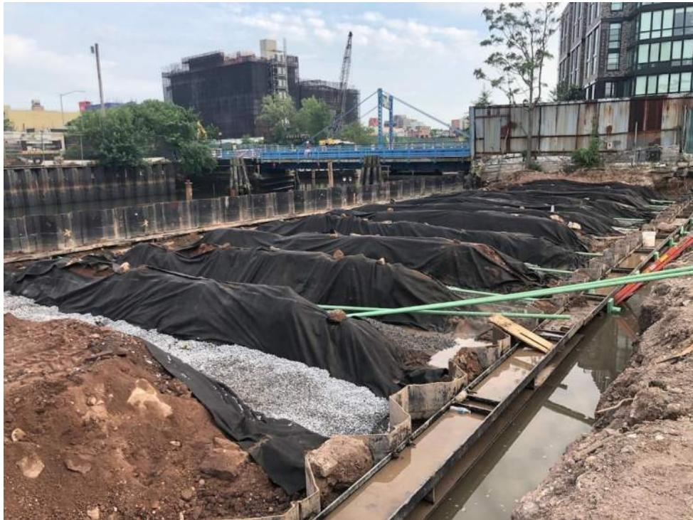
Photo 2: View of tie rod installation, trench excavation, and backfilling progress in the southern region of the site (facing south).
