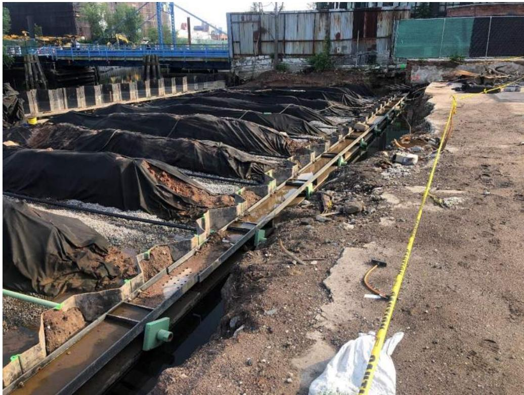
Photo 1: View of tie rods with corrosion protection tape applied (facing south).
