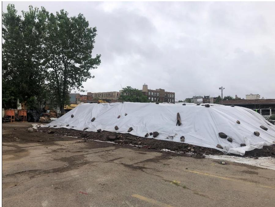
Photo 1: View of covered soil/fill stockpile in Lot 3 at the end of the day (facing northeast).
