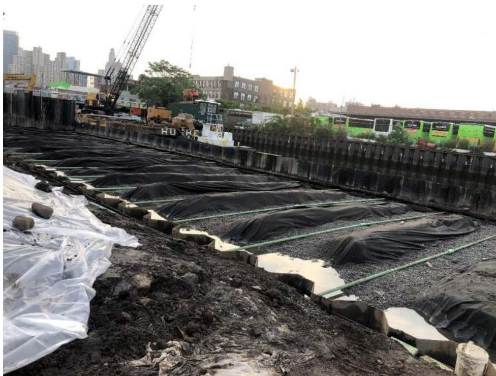
Photo 1: View of tie rod installation progress in the northern region of the site (facing northeast).
