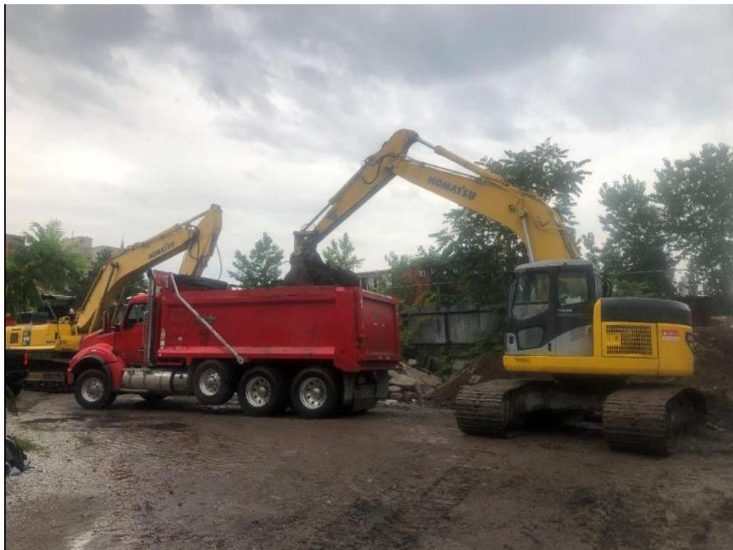
Photo 1: View of A-Construction loading permitted tri-axle truck with non-hazardous soil/fill for off-site disposal (facing north).
