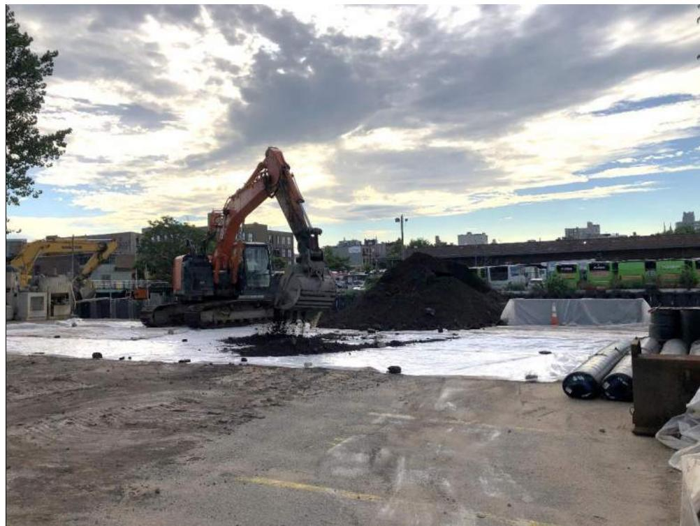
Photo 1: View of stockpile staging area in the northeast region of Lot 3. Soil/fill placed on poly sheeting (facing east).
