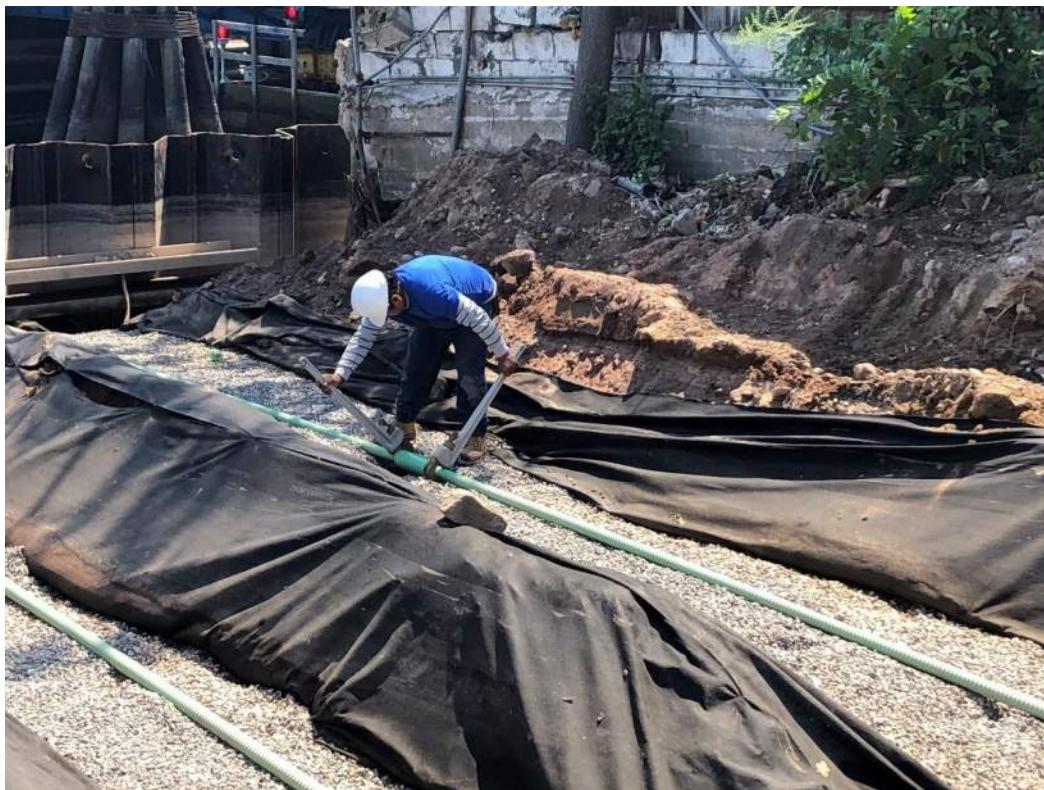
Photo 1: View of Maspeth Masonry tightening the tie rod couplers (facing southeast).
