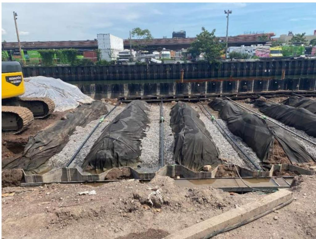
Photo 1: View of tie rods with corrosion protection tape applied (facing east).
