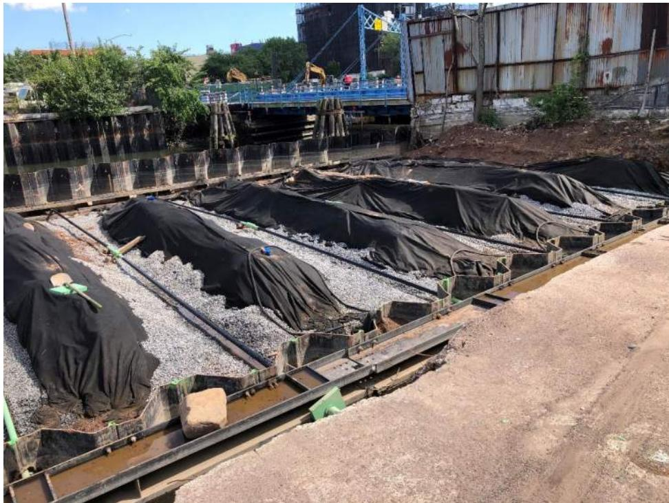
Photo 1: View of tie rods with corrosion protection tape applied (facing southeast).
