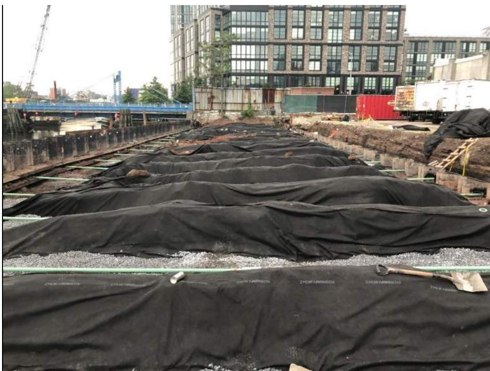
Photo 1: View of tie rod installation, trench excavation, and backfilling progress in the southern region of the site (facing south).
