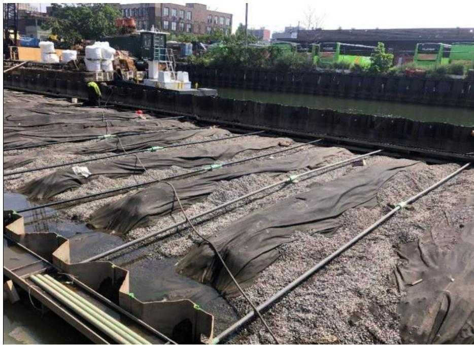
Photo 1: View of tie rods with corrosion protection tape applied (facing north).
