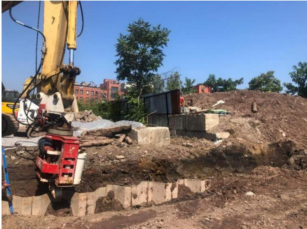
Photo 2: View of use of vibratory hammer working to adjust the height of deadman sheet piles (facing northwest).
