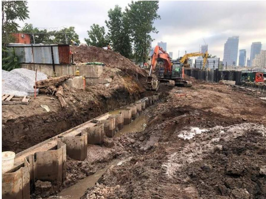
Photo 2: View of sheet pile deadman and steel wale installation progress in the northeast region of the site (facing north).
