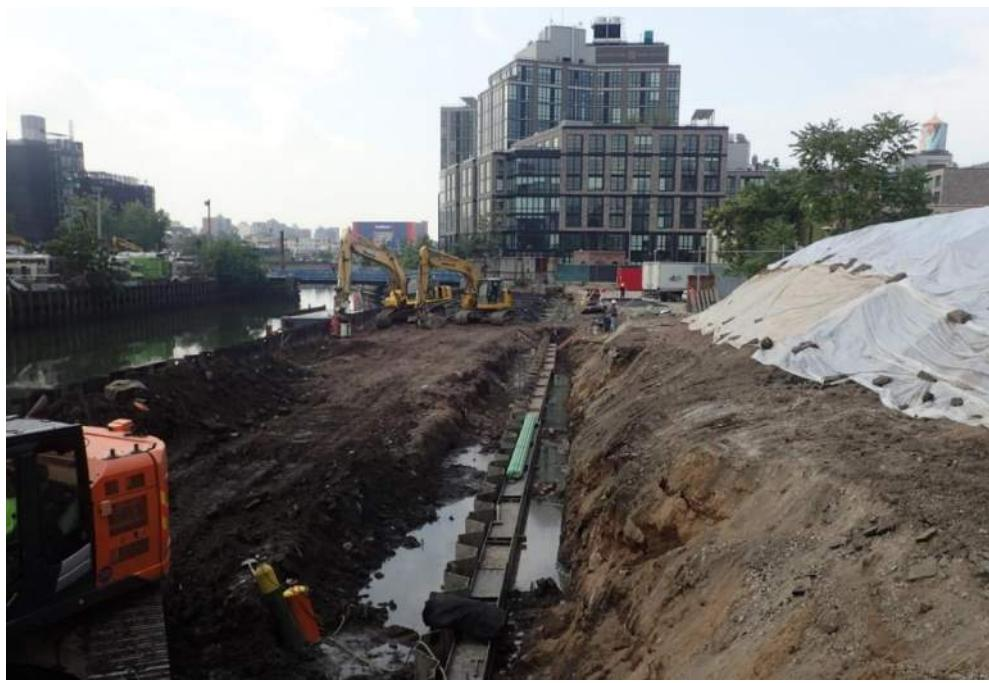
Photo 1: View of wale installation progress along the deadman (facing south).
