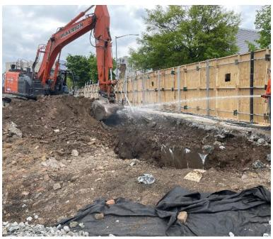
**Photo 1:** Mayrich excavating former foundation elements and spraying water to control dust in the southeastern portion of BCP Site No. C224309
