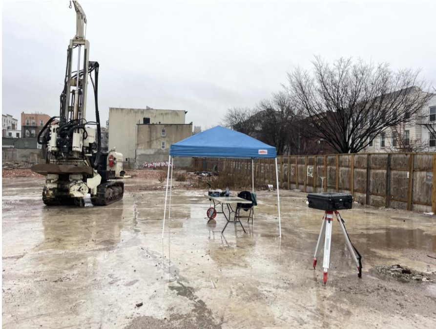
Photo 1: Eastern Environmental advancing soil boring SB03_CT in the central part of 473 President Street (facing southeast)
