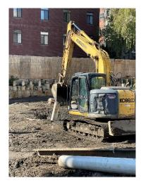
Photo 3: Excavation and installing new suction point in the middle of the site.
