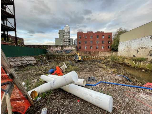
Photo 1: Pre-work view of the site facing west.
