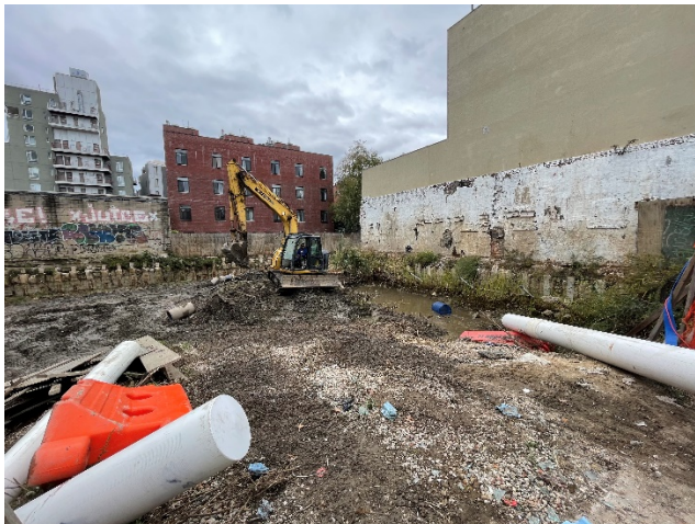
Photo 3: Post-work view of the site facing west.
