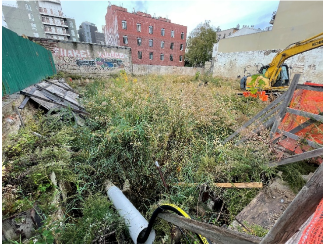
Photo 1: Pre-work view of the site facing northwest.
