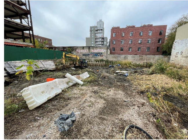
Photo 2: View of the site after vegetation removal.
