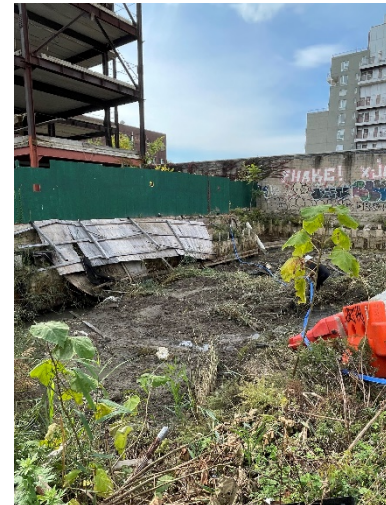
Photo 4: View newly installed dewatering suction points.
