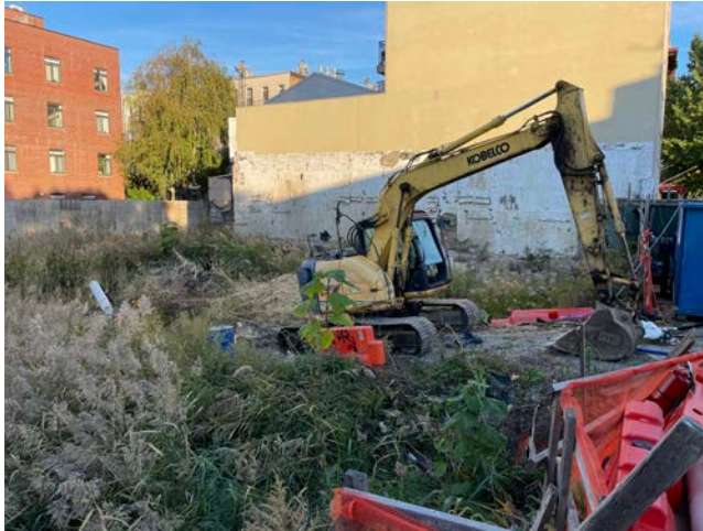
Photo 1: Pre-work view of the site facing northeast.
