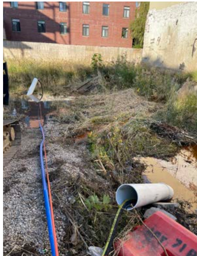
Photo 3: View of dewatering suction points.
