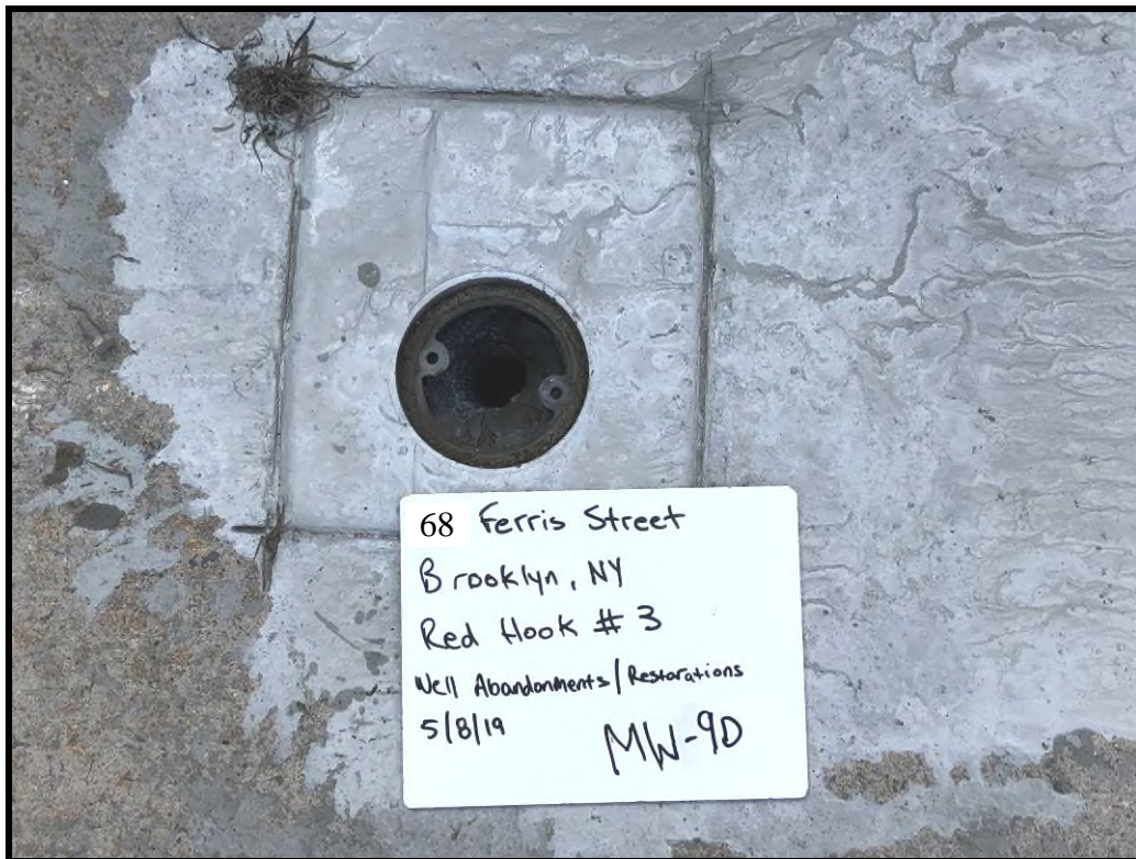
MW-9D with PVC Riser Grouted
