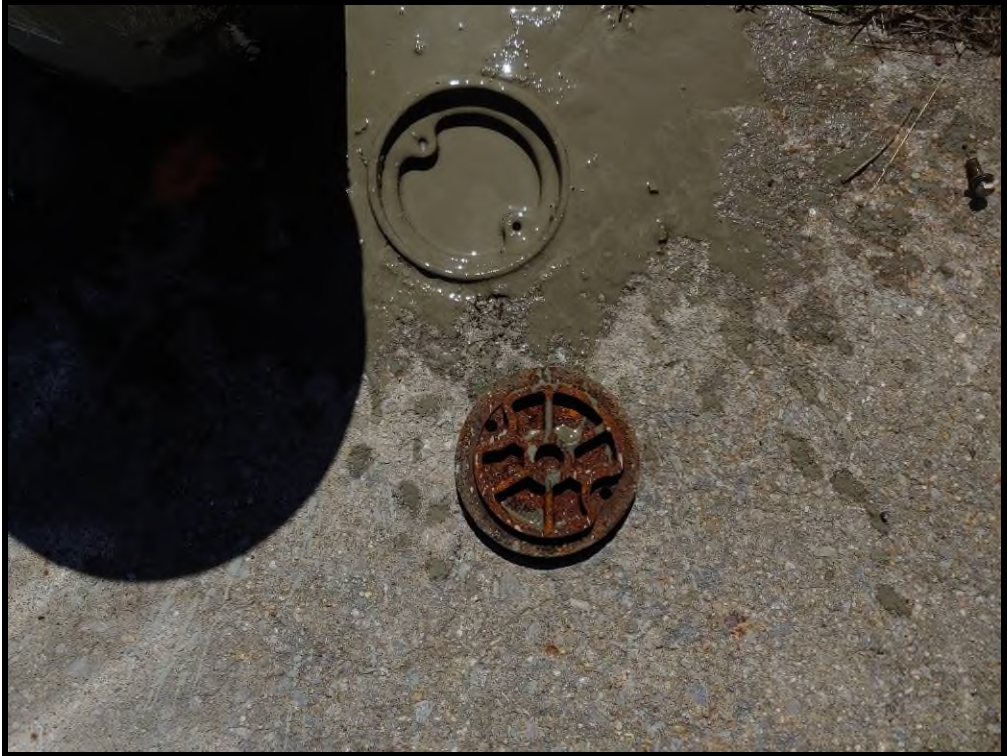
TMW-1 with PVC Riser Grouted
