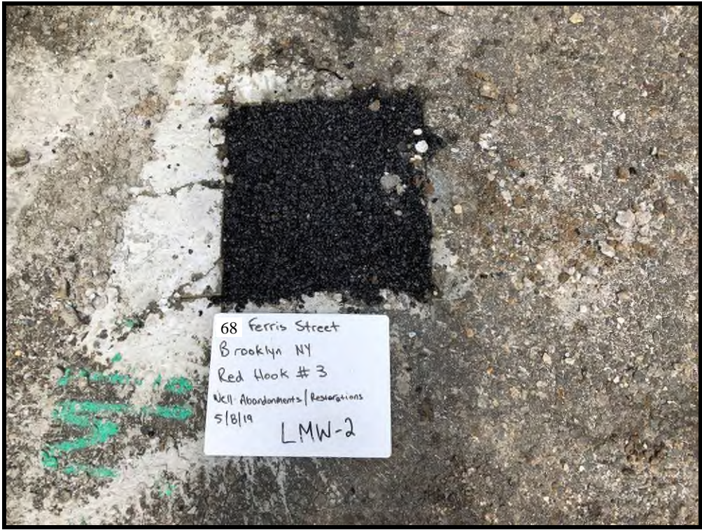
LMW-2 Surface Completion
