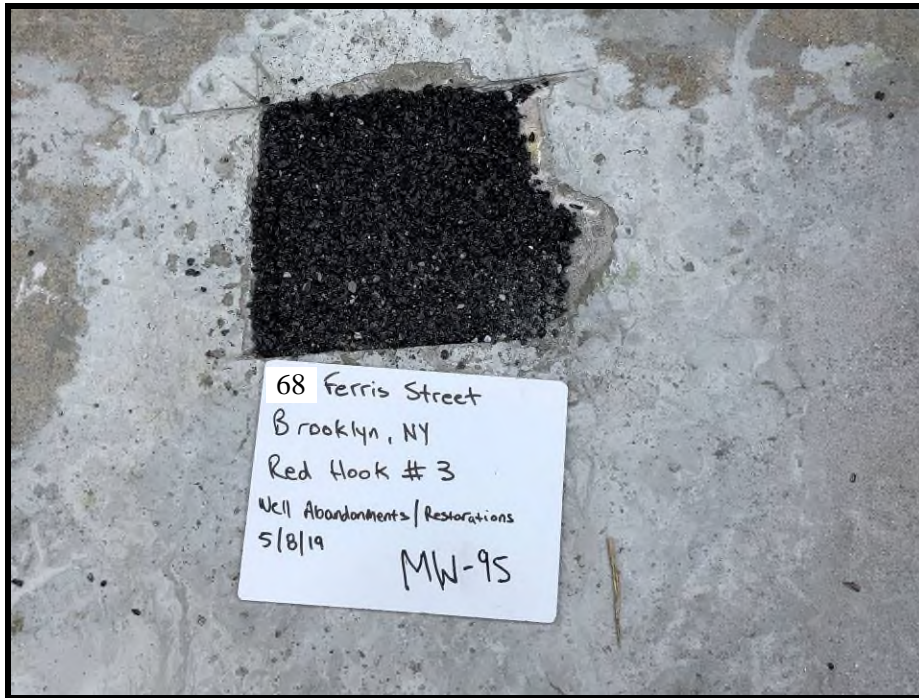
MW-9S Surface Completion with Cold Patch
