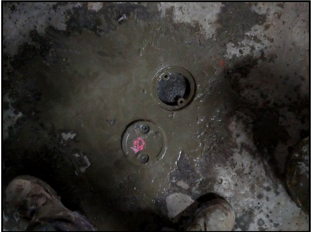
LMW-8S (Inside Blue Warehouse) with PVC Riser Grouted
