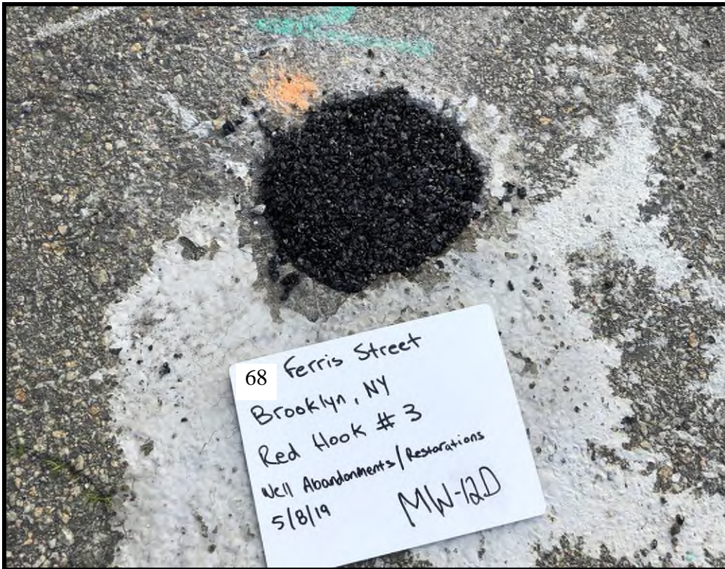
MW-12D Surface Completion with Cold Patch
