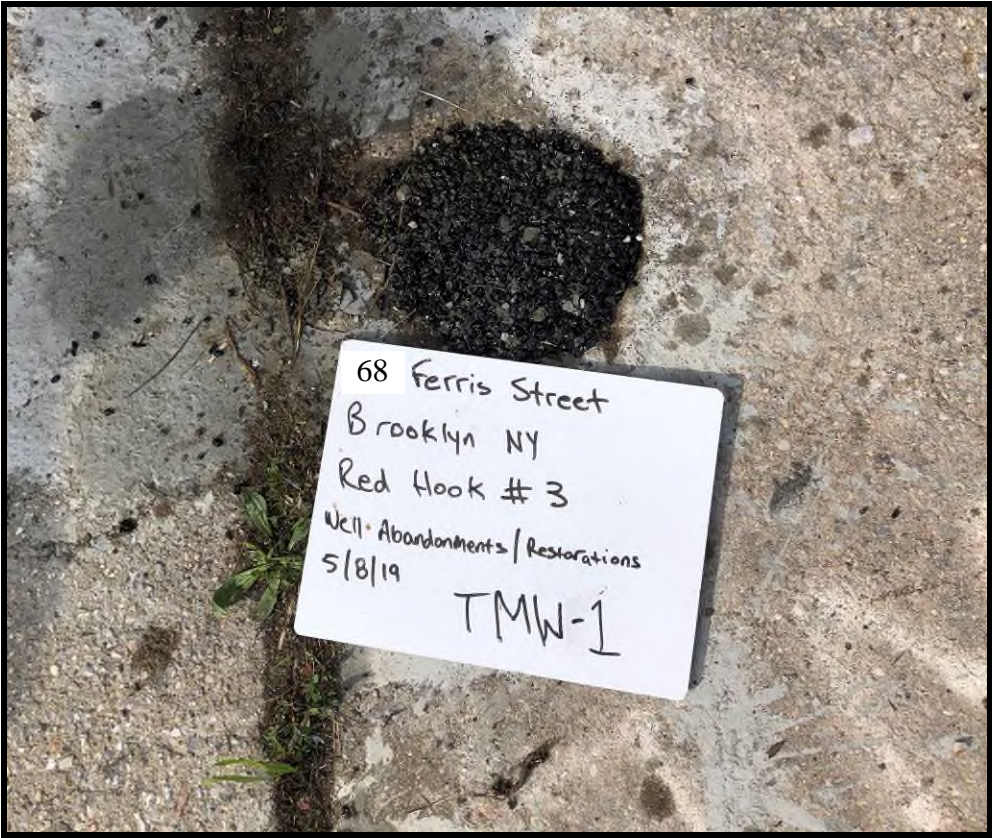
TMW-1 Surface Completion with Cold Patch
