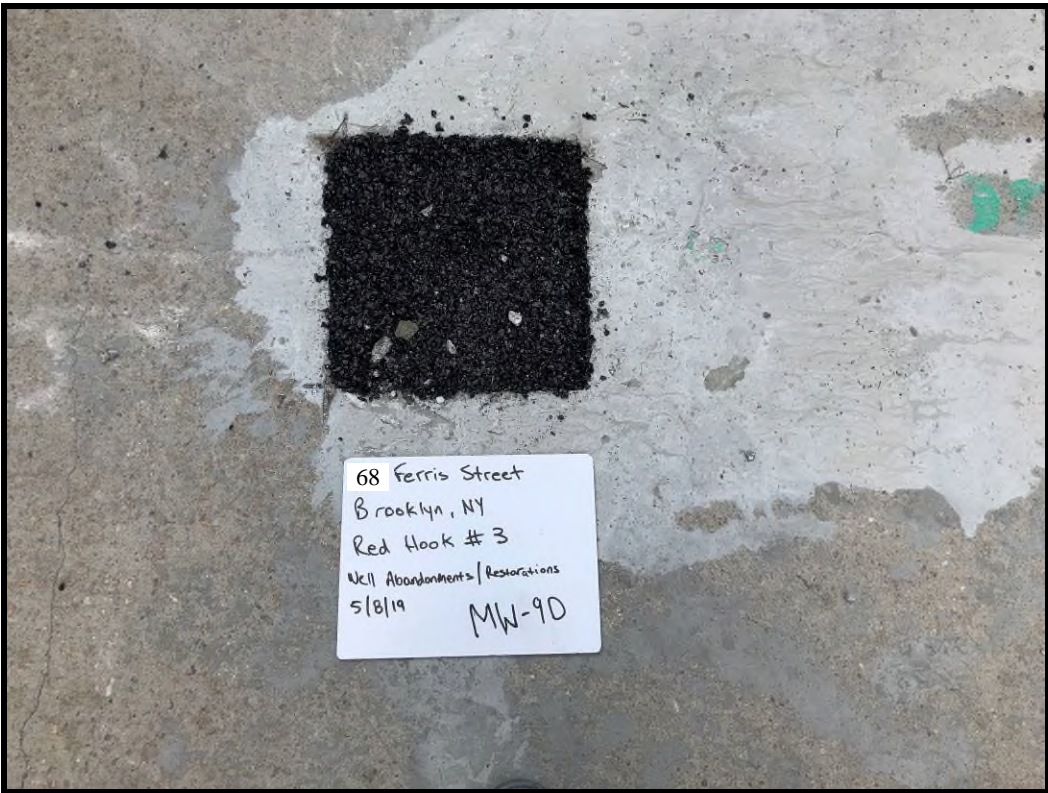
MW-9D Surface Completion with Cold Patch
