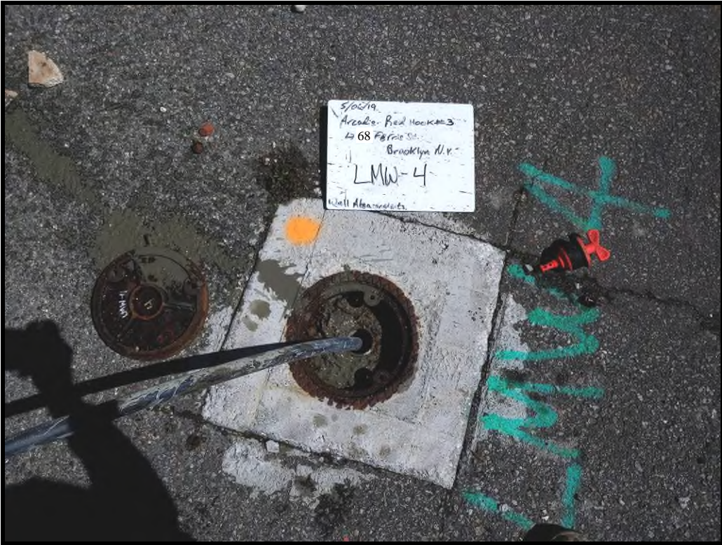
LMW-4 PVC Screen and Riser in Process of Grouting (Typical)
