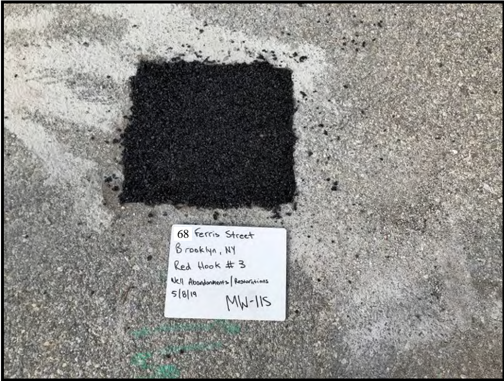
MW-11S Surface Completion with Cold Patch
