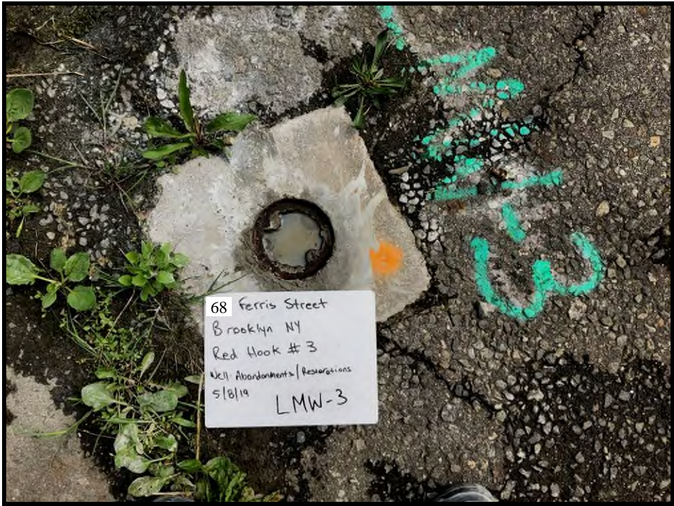
LMW-3 with PVC Riser Grouted
