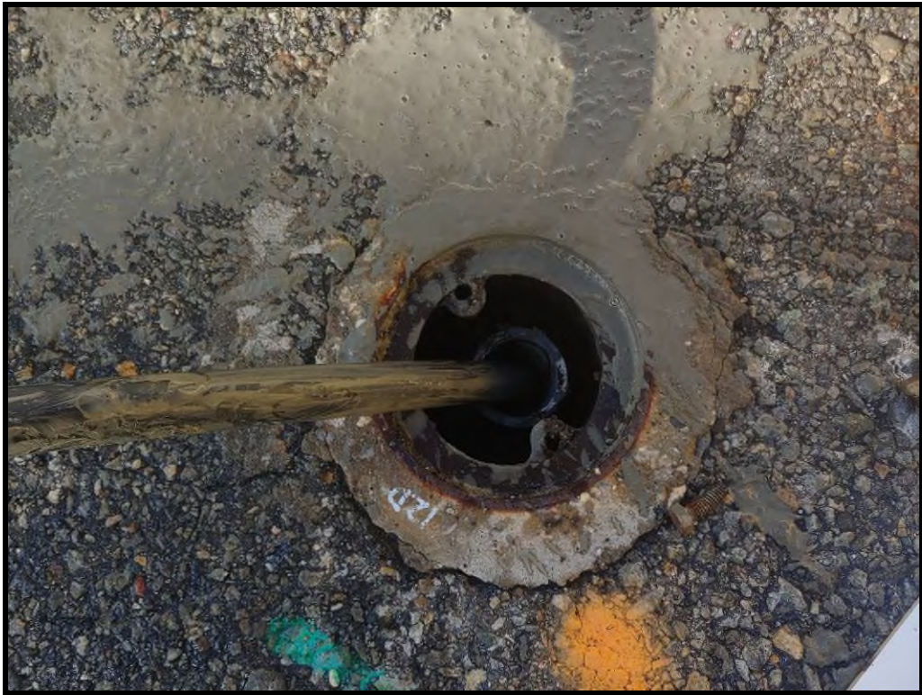
MW-12D with PVC Screen and Riser in Process of Grouting
