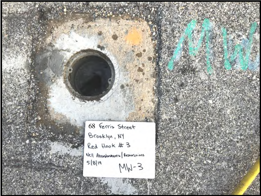
MW-3 with PVC Riser Grouted
