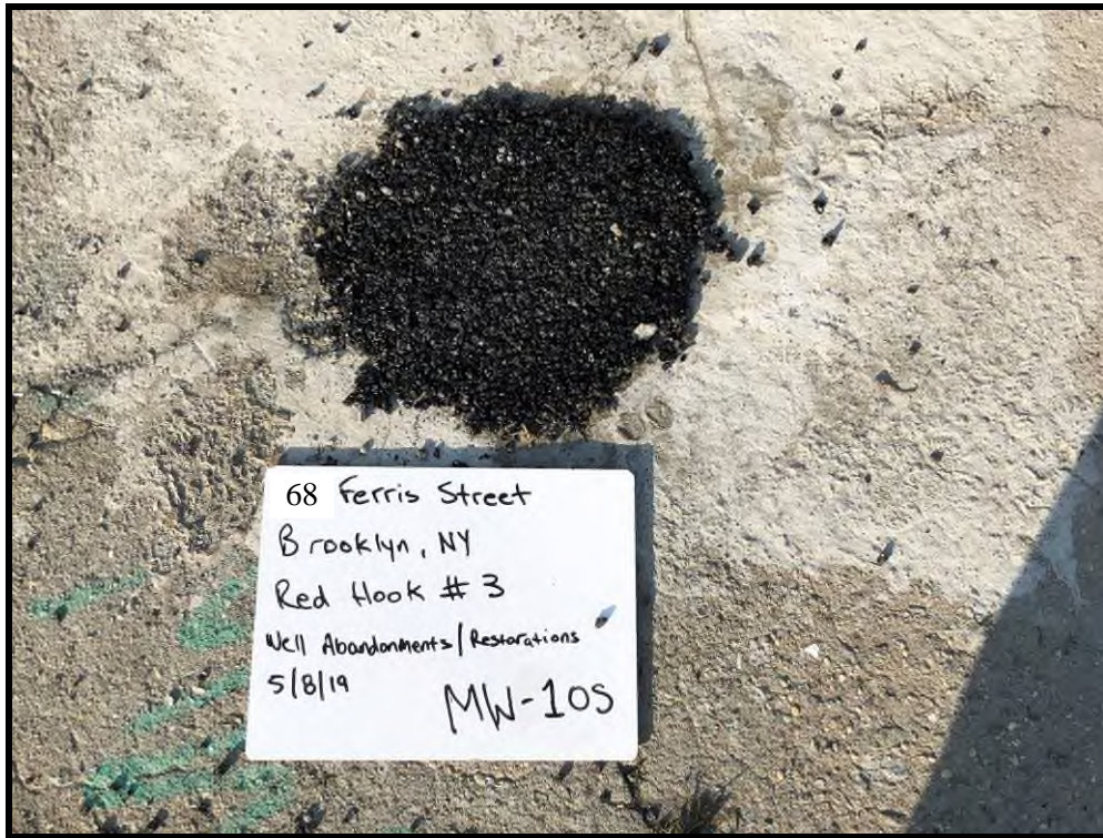
MW-10S Surface Completion with Cold Patch
