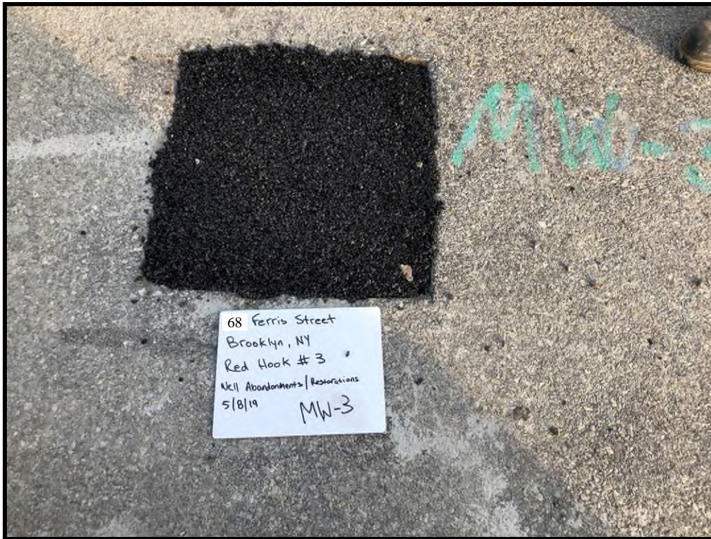
MW-3 Surface Completion with Cold Patch
