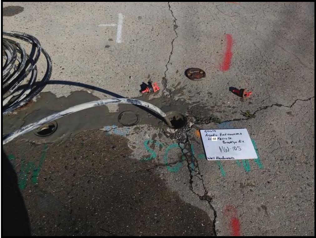
MW-10S with PVC Screen and Riser in Process of Grouting
