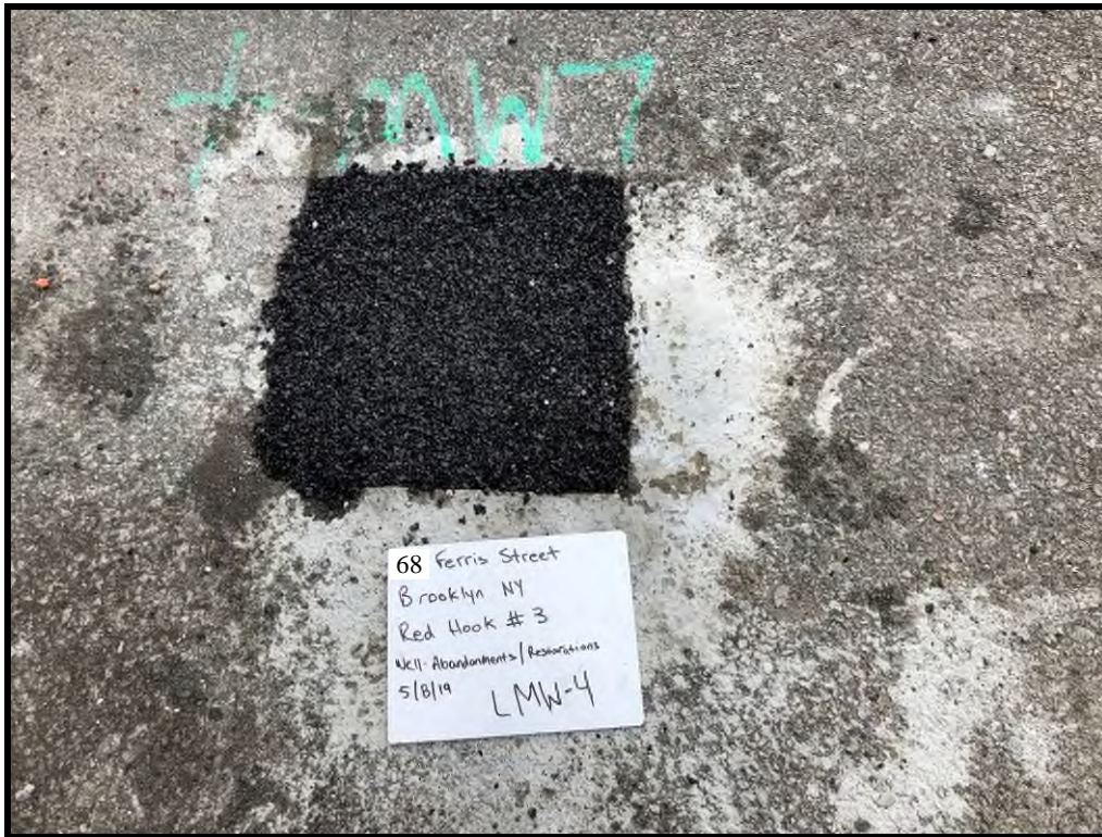
LMW-4 Surface Completion with Cold-Patch
