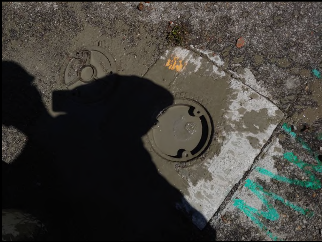
LMW-4 with PVC Riser Grouted
