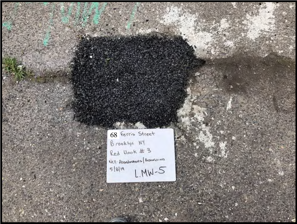
LMW-5 Surface Completion with Cold-Patch
