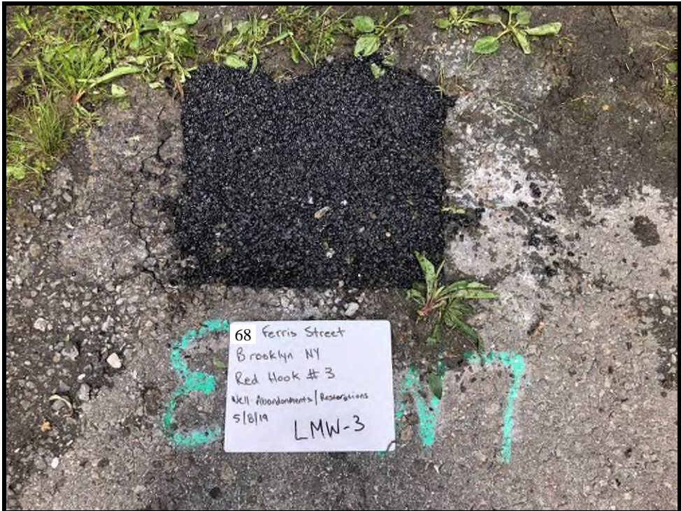
LMW-3 Surface Completion with Cold-Patch
