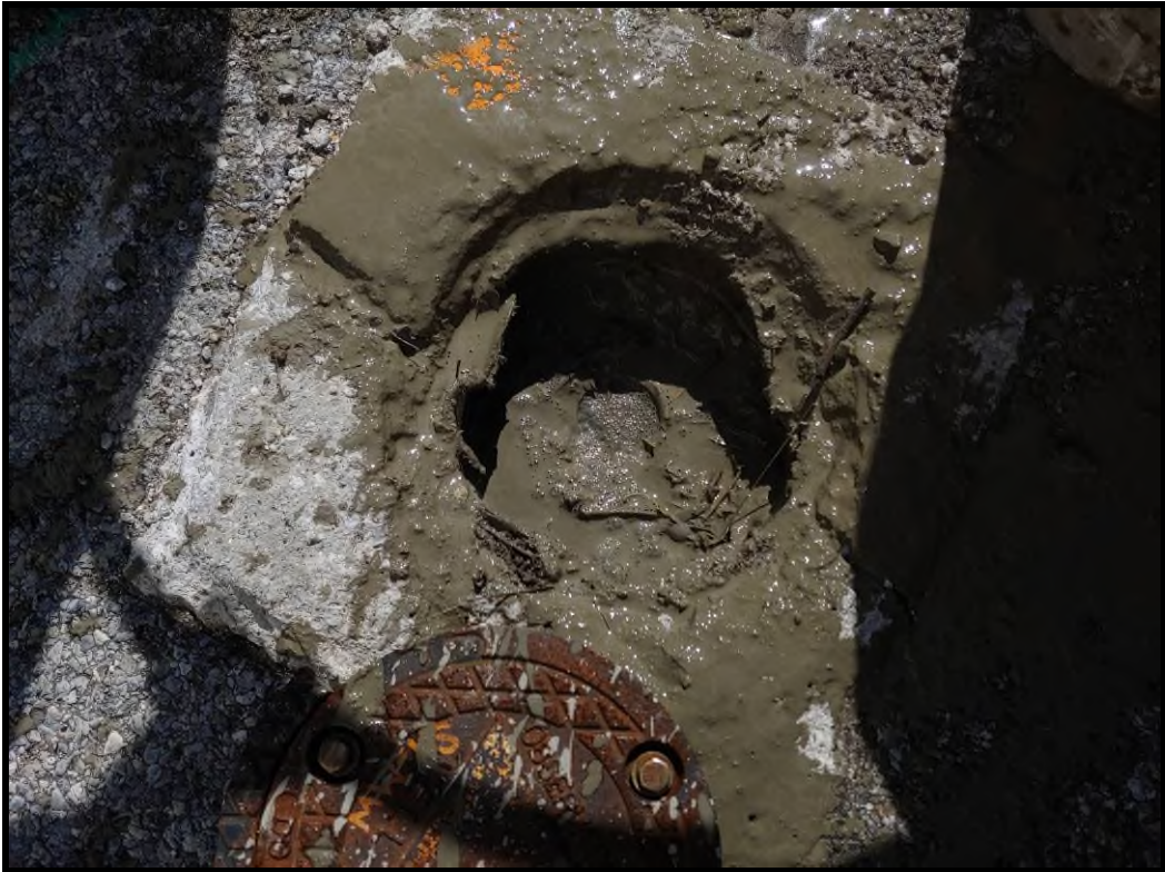
MW-11S with PVC Riser Grouted
