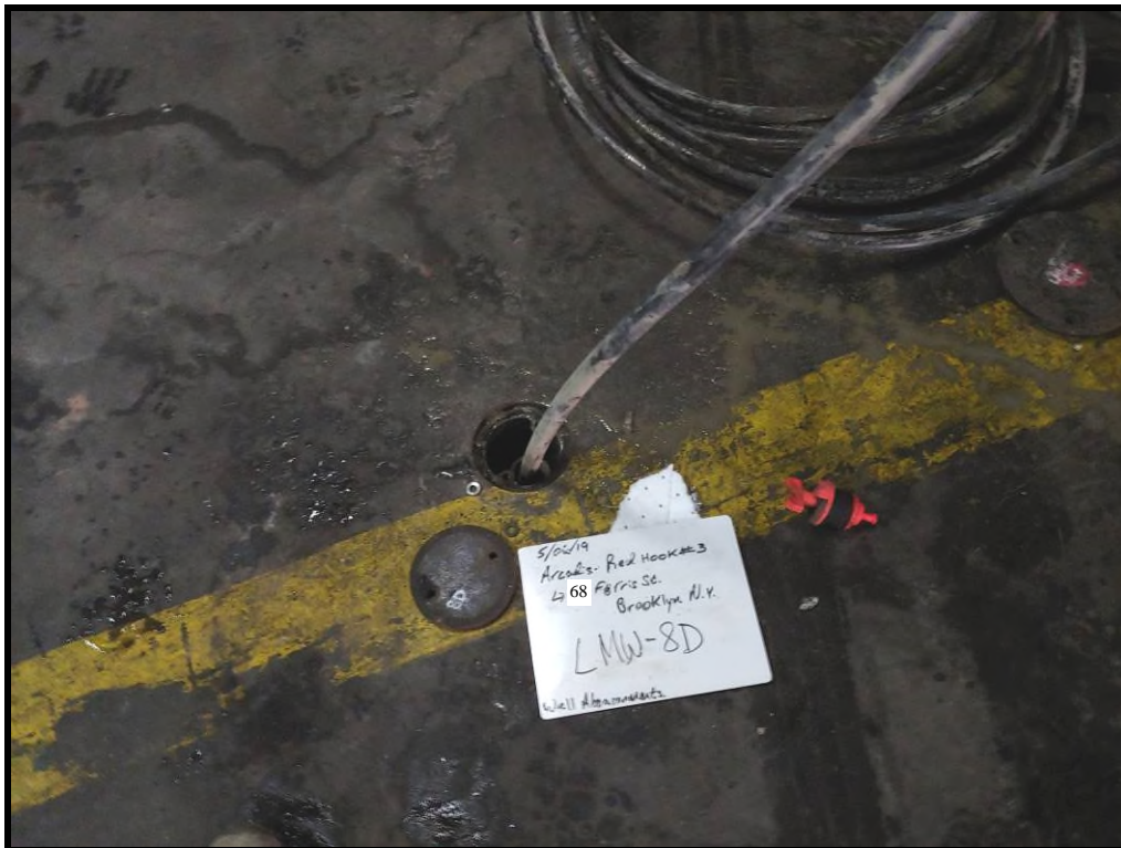
LMW-8D (Inside Blue Warehouse) with Grouting in Progress
