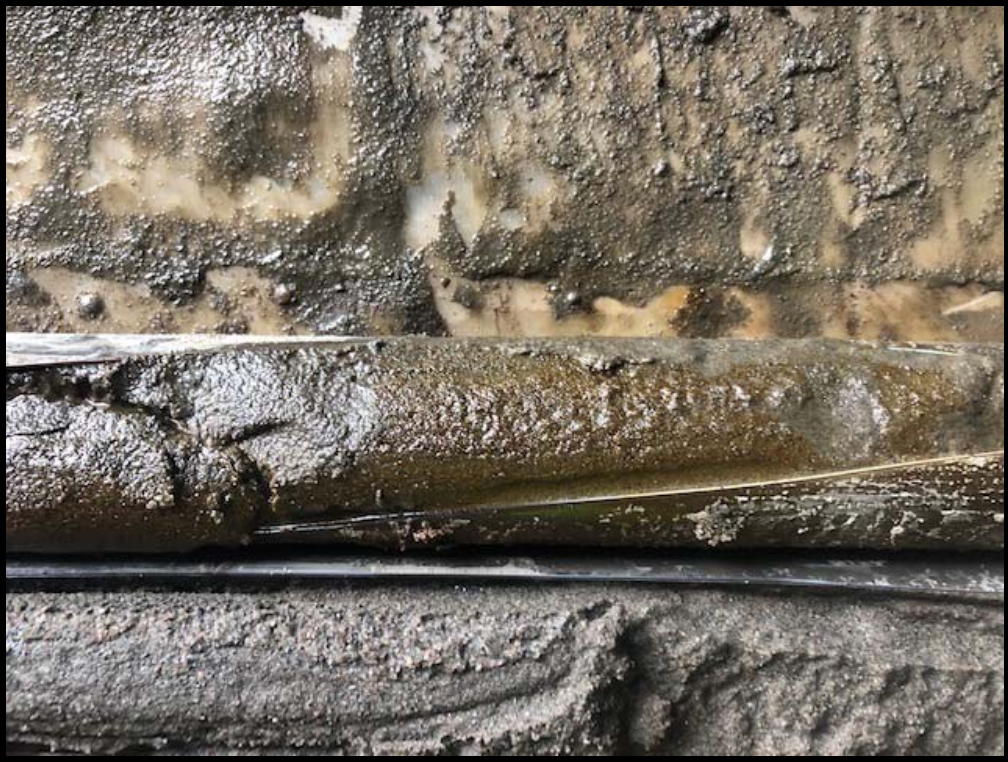
A-RH3-WS16: Close-up of Staining in 20- to 25-Foot Interval
