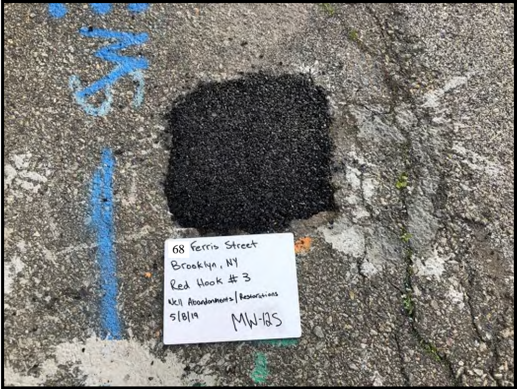
MW-12S Surface Completion with Cold Patch
