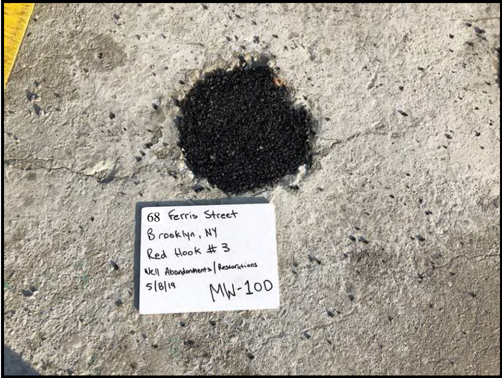
MW-10D Surface Completion with Cold Patch
