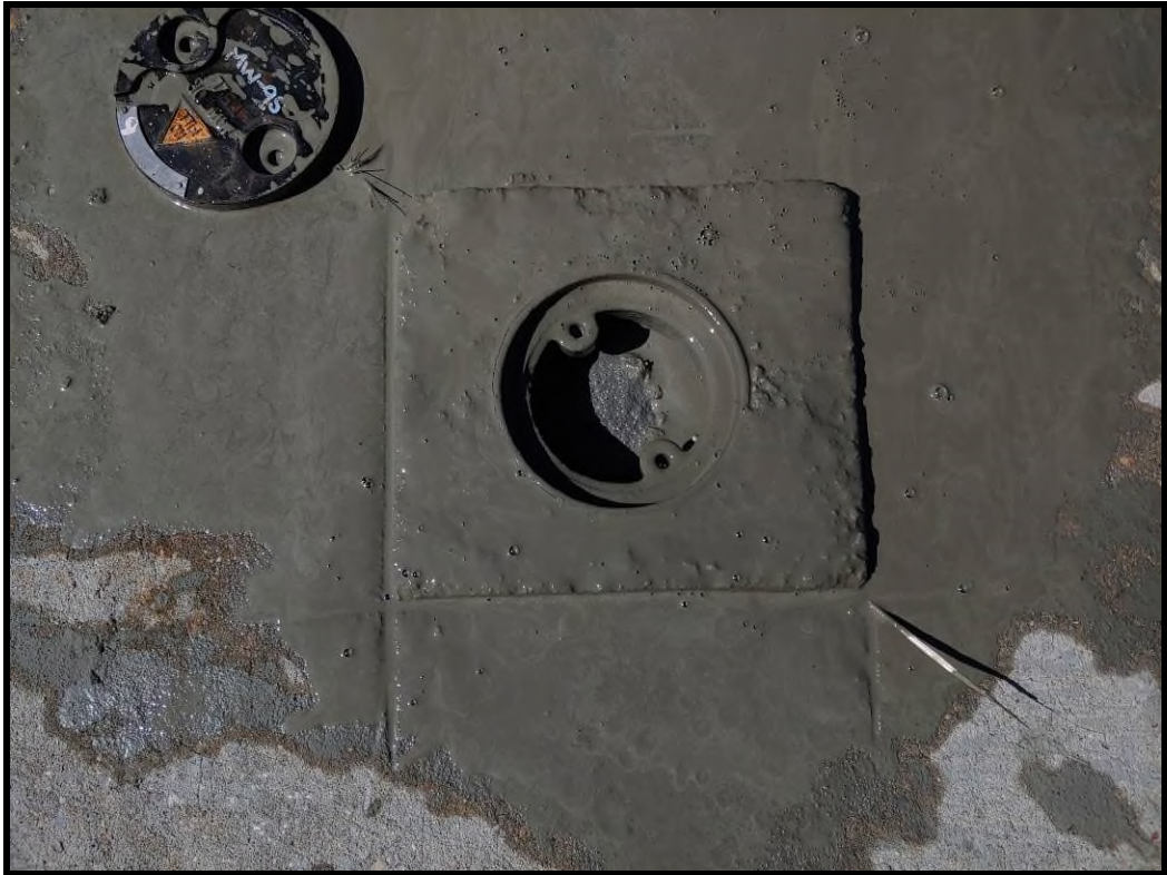
MW-9S with PVC Riser Grouted
