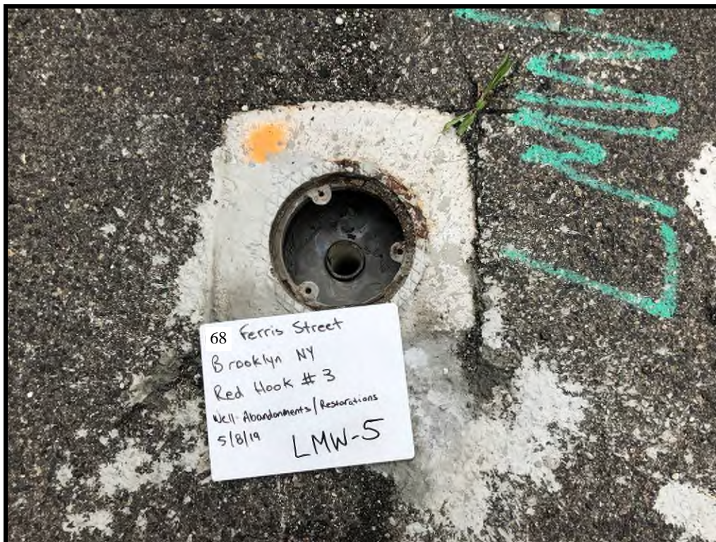
LMW-5 with PVC Riser Grouted
