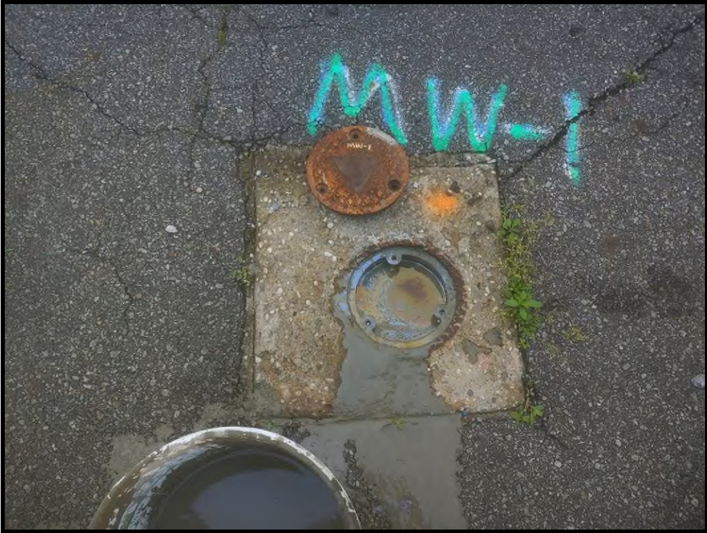
MW-1 with PVC Riser Grouted
