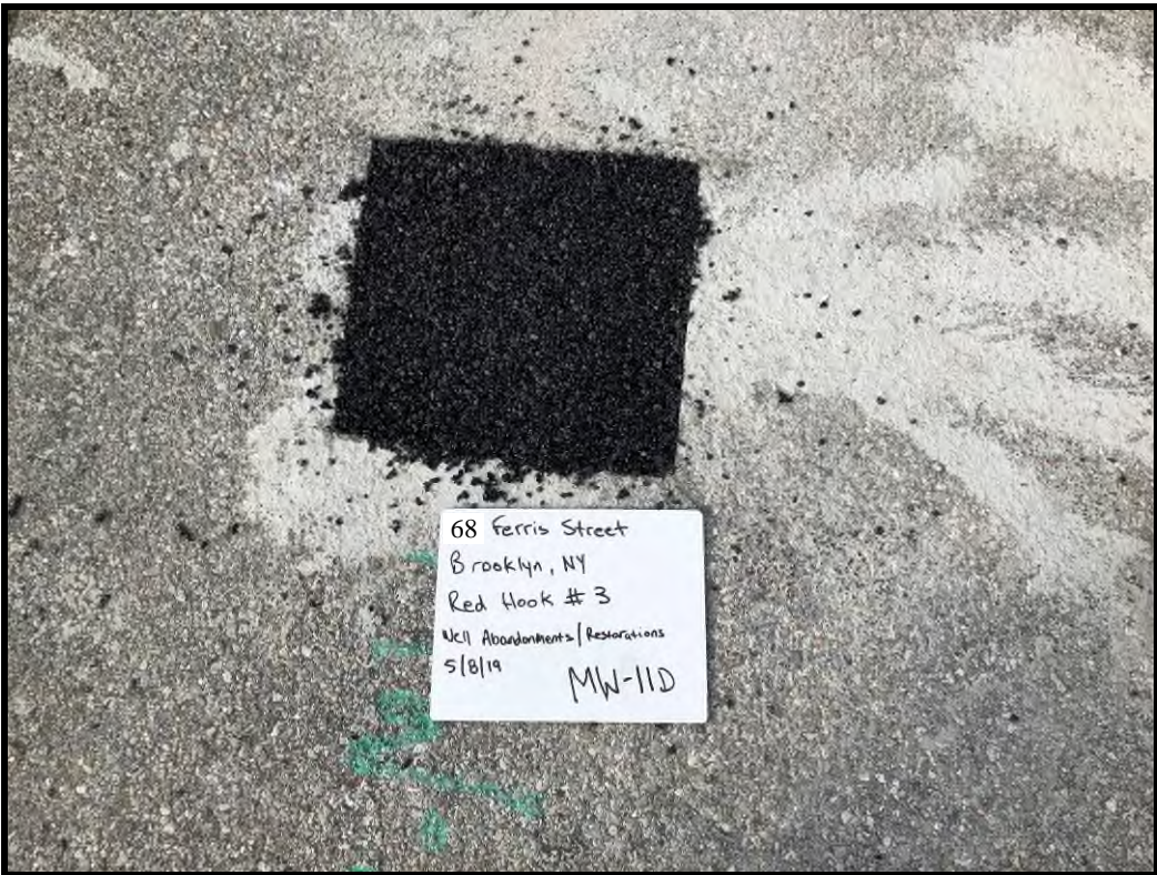
MW-11D Surface Completion with Cold Patch
