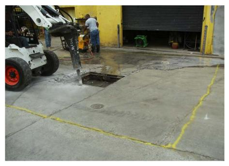
1. Concrete being broken around the former sediment trap. The yellow line shows the extent of the excavation.
