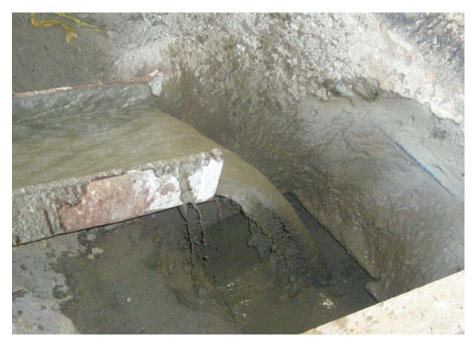
8. 3,000-gallon UST being filled with concrete slurry
