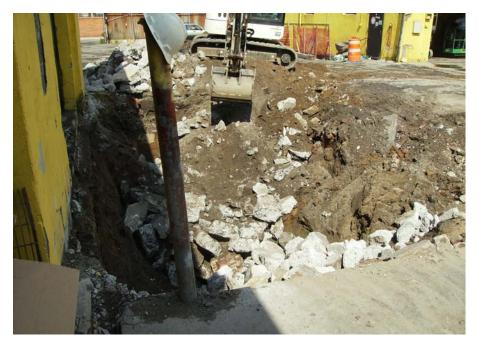
3. Excavation of contaminated soil immediately east of machine shop.
