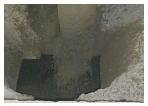
7. 3,000-gallon UST being filled with concrete slurry
