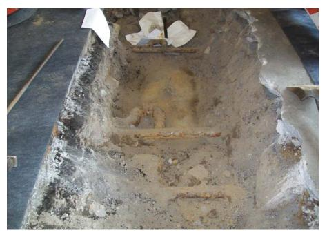
5. Top of 3,000-gallon UST exposed beneath floor of machine shop.
