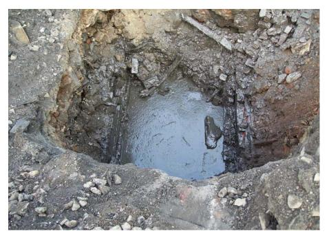
1. Excavations immediately beneath monitoring well BK-10 revealed the presence of a brick-lined channel containing grossly contaminated soil at 7 feet below surface grade.
