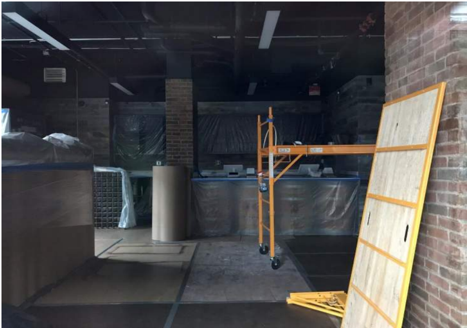
Photo 19: Commercial space in southwest portion of the building, facing north. 6 February 2020.
