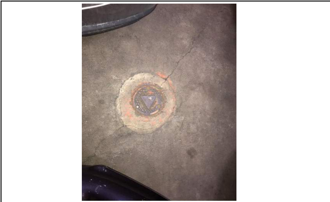
Photo 4: Groundwater monitoring well (PMW-4) within subgrade parking area, facing north. 6 February 2020.
