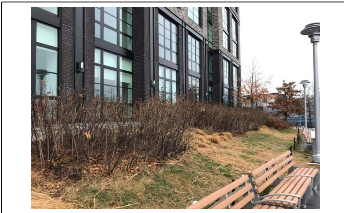
Photo 16: Paved and landscaped esplanade areas, facing north. 6 February 2020.
