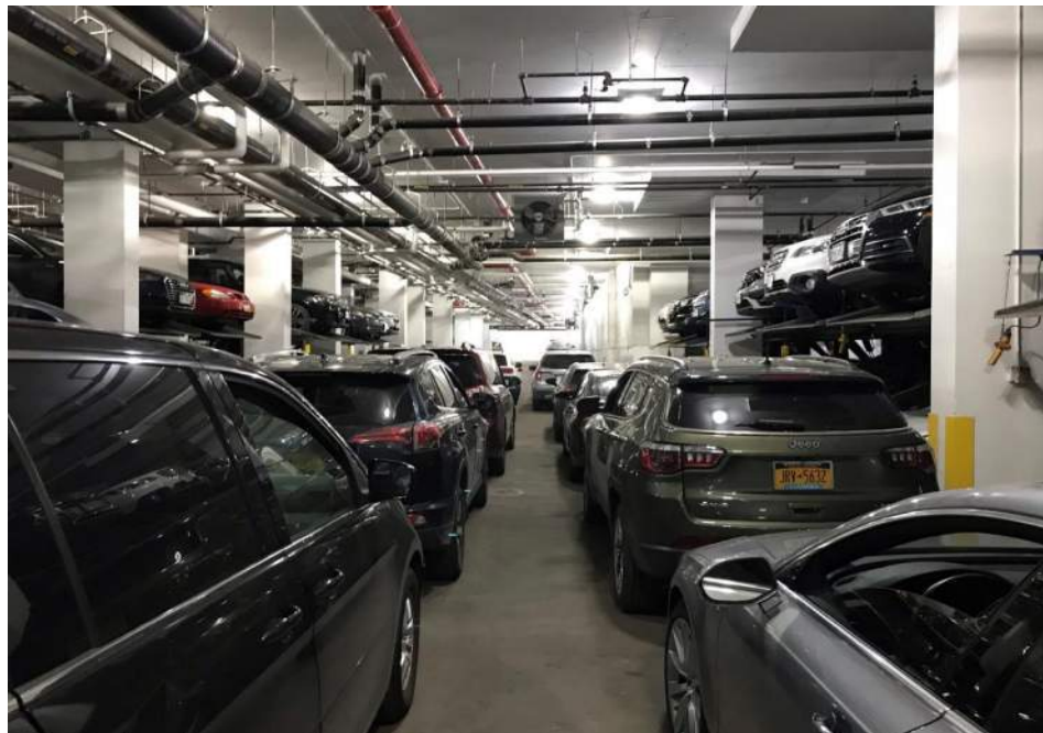
Photo 2: Subgrade parking lot concrete slab, facing west. 21 April 2021.
