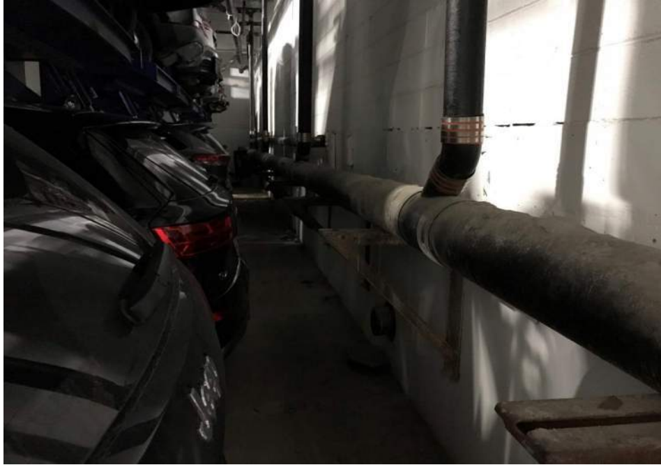
Photo 5: Subgrade parking lot concrete foundation wall (beneath the first floor), facing northwest. 21 April 2021.
