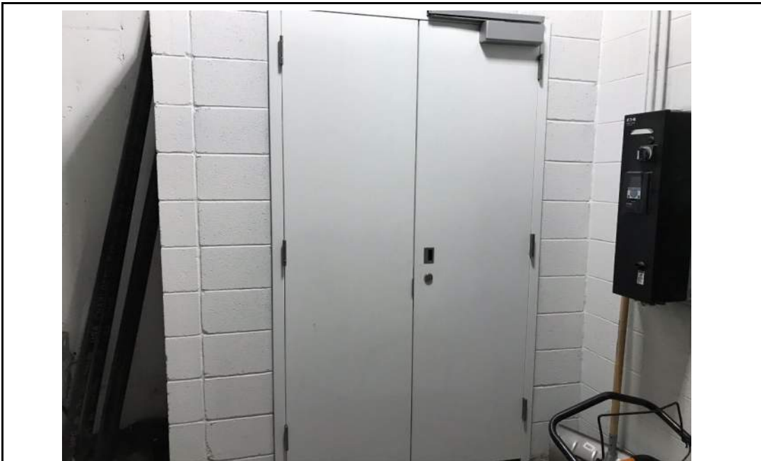
Photo 6: Air Sparge/Soil Vapor Extraction (AS/SVE) manifold closet within subgrade parking area, facing west. 6 February 2020.
