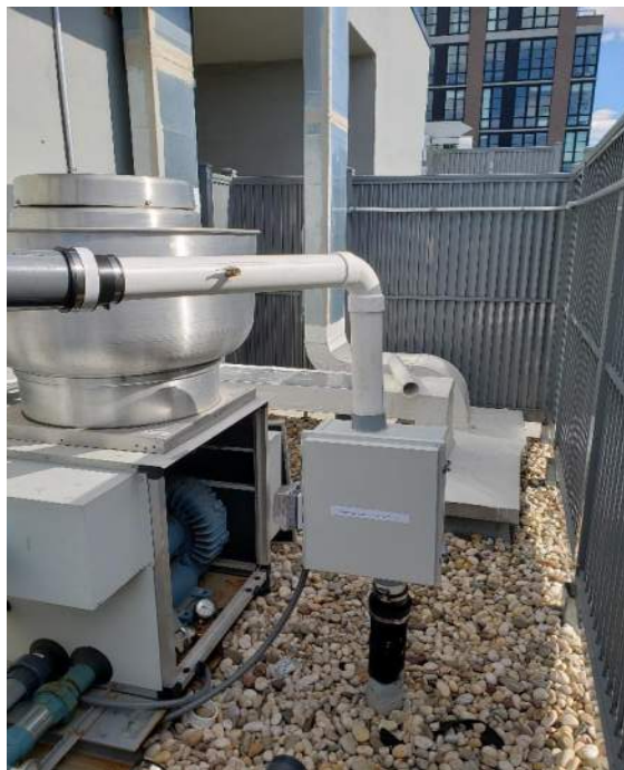
Photo 5: Installation of new Obar fan at V1 location. 8 October 2020.
