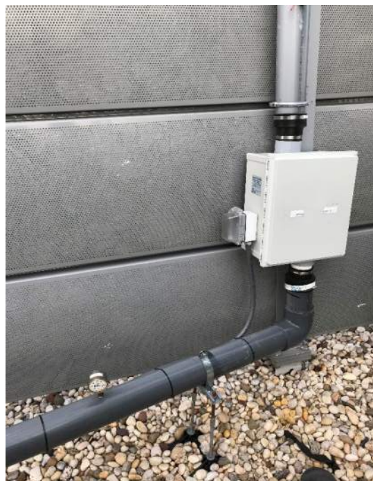
Photo 7: New Obar fan at V2 location. 21 April 2021.
