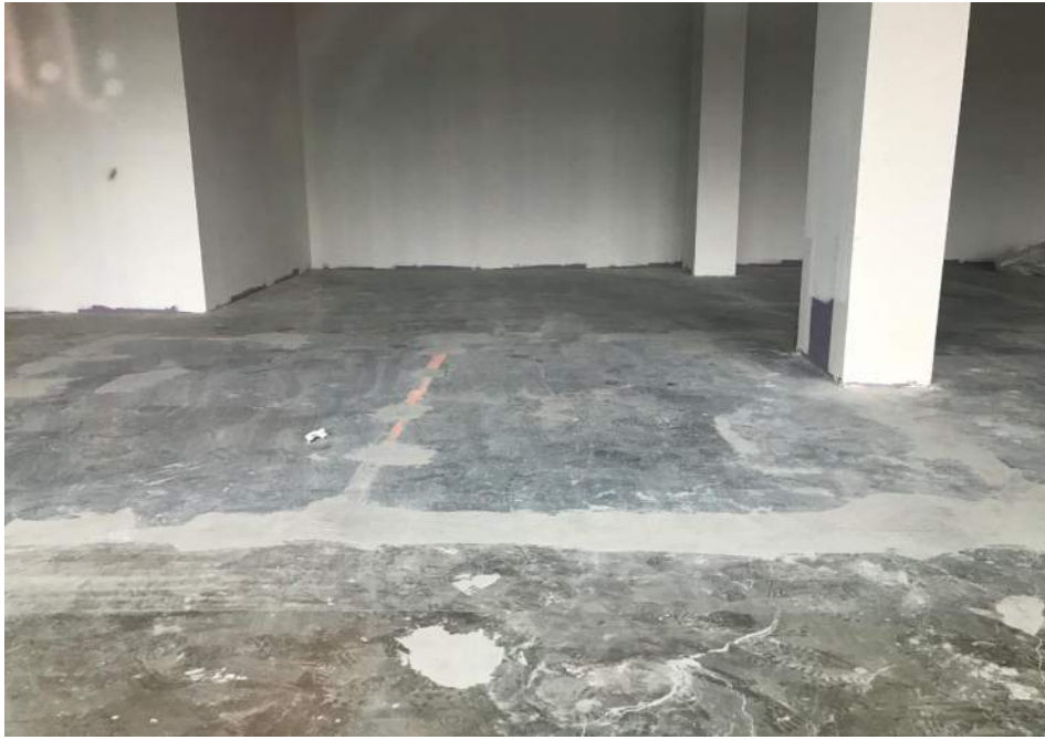
Photo 18: Commercial space in northeast portion of the building, facing south. 6 February 2020.
