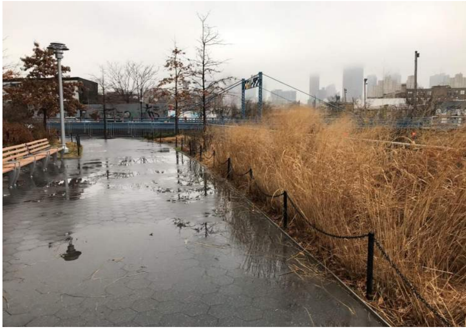
Photo 17: Paved and landscaped esplanade areas, facing east. 6 February 2020.
