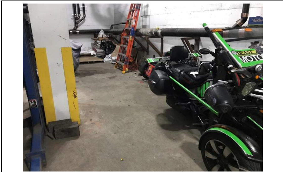
Photo 3: Subgrade parking lot concrete slab, facing east. 21 April 2021.
