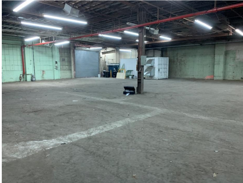
Photo 1: General view of Site cover system (facing northwest)
