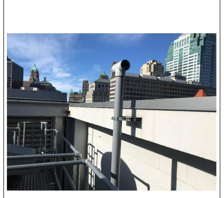
Photo 8: SVE system exhaust stack
