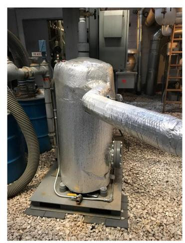
Photo 5: SVE inlet piping to knockout tank
