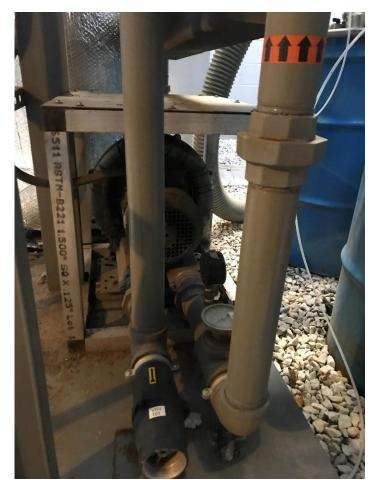
Photo 6: SVE blower inlet and outlet piping
