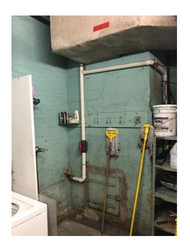
Photo 10: SJHS SSDS piping in boiler room and extraction point
