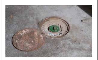
Photo 7: Groundwater monitoring well
