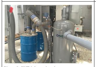
Photo 5: SVE inlet and moisture separator
