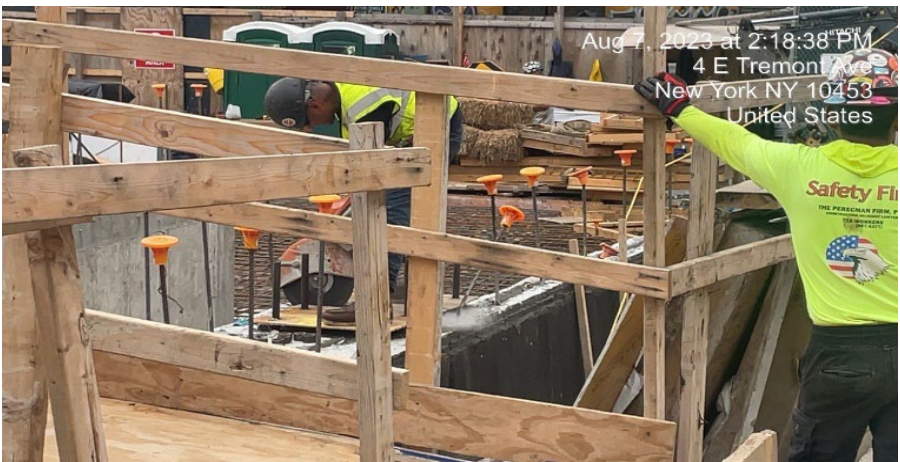
Photograph 3 - Workers cutting metal in preparation for steel installation. View facing northwest.
