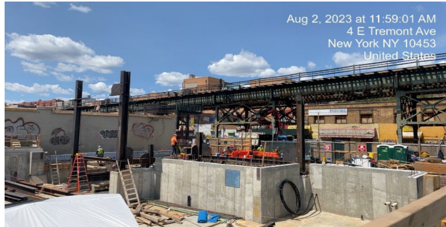
Photograph 2 - Metal work being done in WC-03. View facing northwest.
