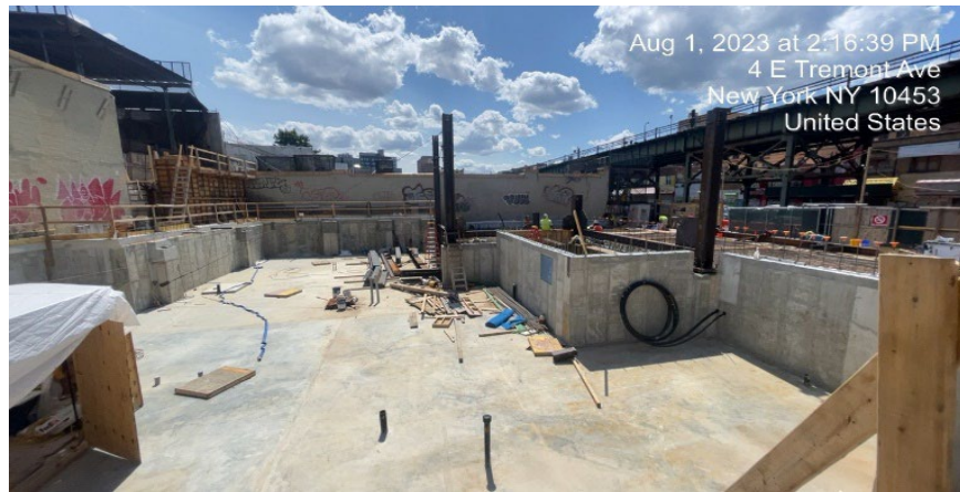
Photograph 3 - A view of the Site facing south.
