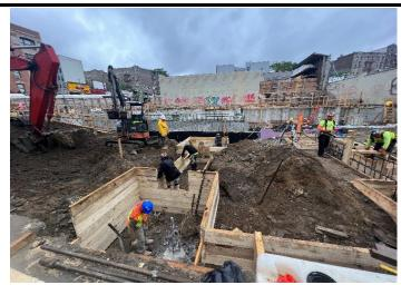
Photograph 3 - Site condition. Casino installing rebar in WC 01. View facing Northeast.
