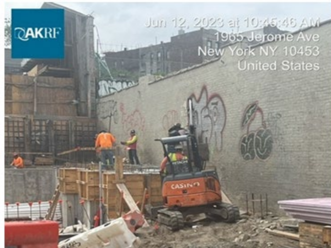
Photograph 3 - Casino working on rebar formwork WC- 03. Facing southwest.
