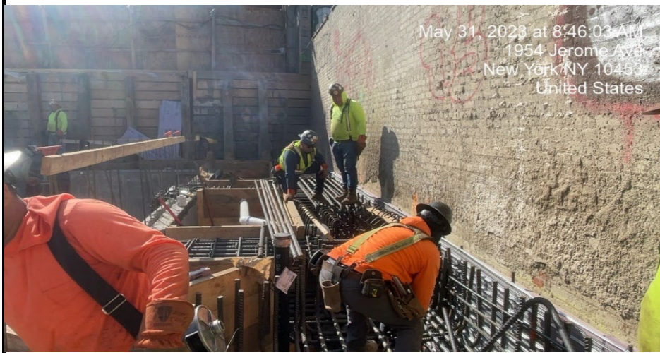
Photograph 1 - The plumbing crew installation SSDS piping in WC-03
