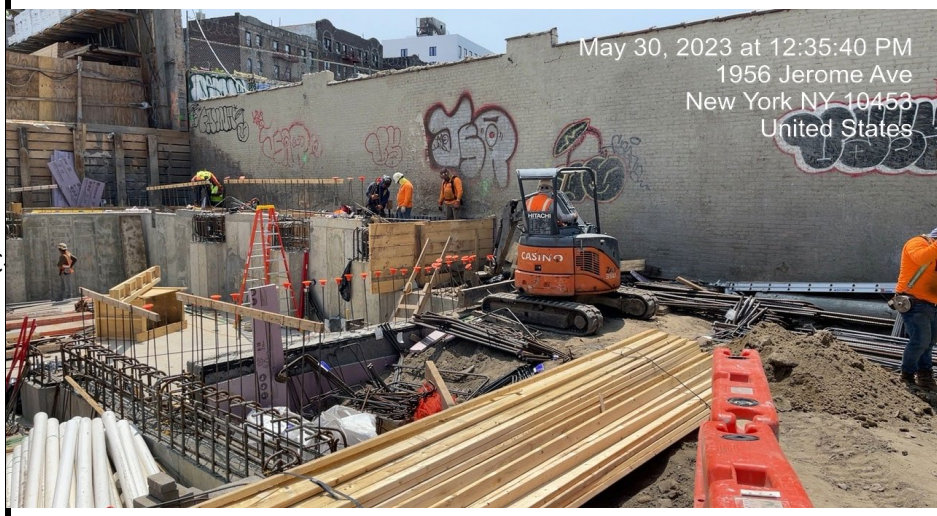
Photograph 3 - Light soil movement in WC 03, facing south east
