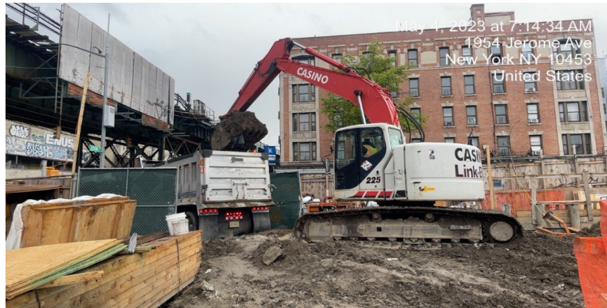
Photograph 1 - Loading a truck for off-site disposal. View facing North.
