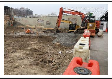
Photograph 3-Excavation of soil against SOE wall in WC-03, view facing south.
