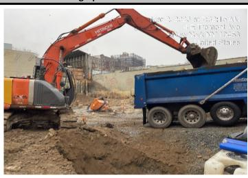
Photograph 2- The excavator spreading 3/4-inch virgin bluestone in WC-02, view facing southwest.
