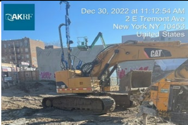
Photograph 2 - The foundation contractor regrading the site, view facing east.
