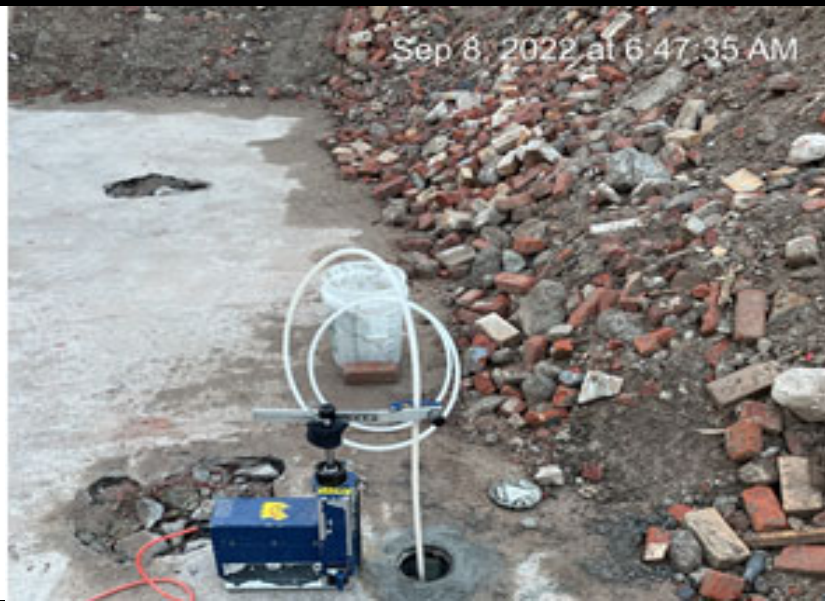
Photograph 1 - The waterra pump set up at RDI-MW-12 to develop the well.
