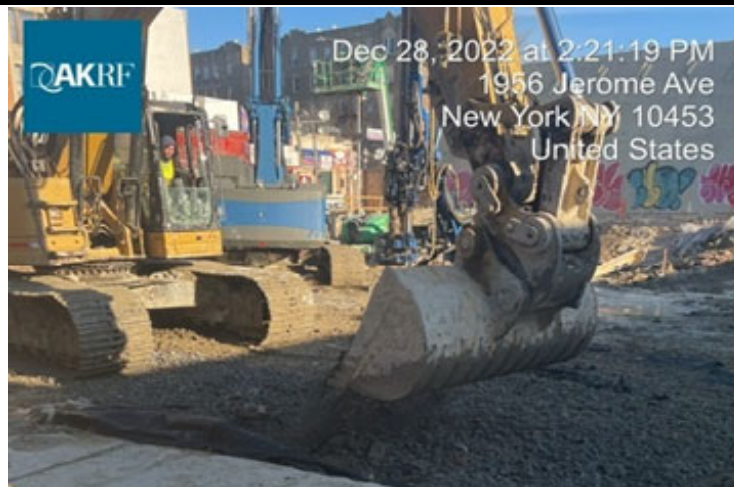
Photograph 3 - The foundation contractor fixing the bluestone truck ramp. View facing east.
