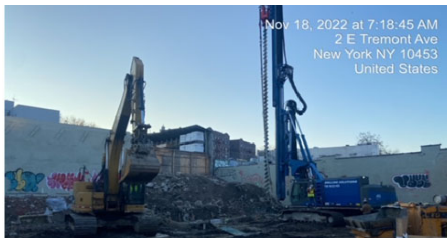
Photograph 3 - the foundation contractor drilling piles in the south of the site.
