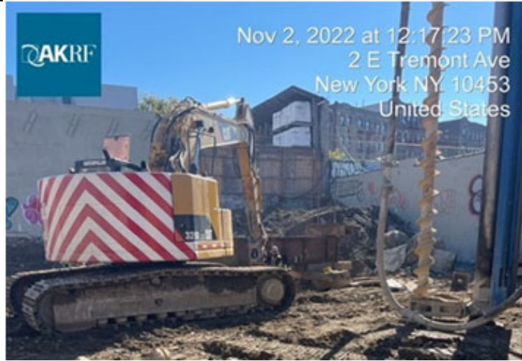
Photograph 1 - the excavation contractor prepping the site for load tests.
