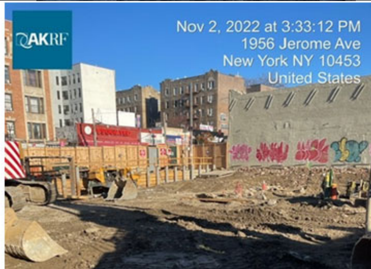
Photograph 3 - Site overview facing northeast.
