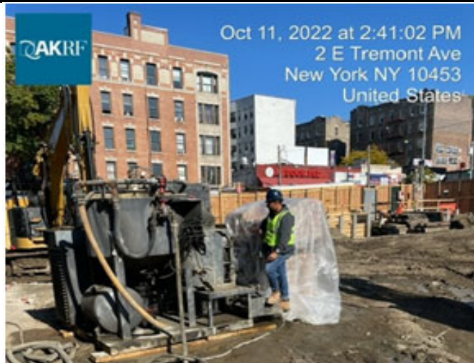
Photograph 2 - Casino grouting piles. View facing east.
