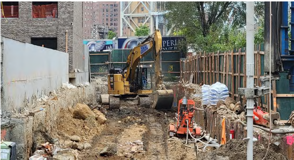
Photograph 3 - Site Grading in Grid A1, view facing northwest.
