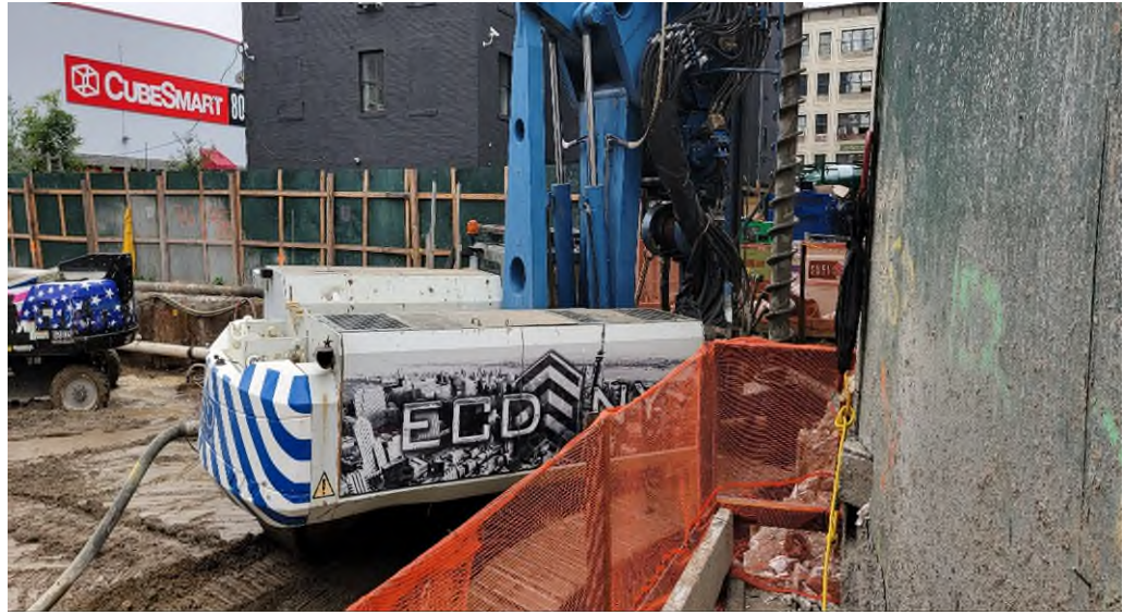
Photograph 1 - ECD drilling piles in Grid A3, view facing east.
