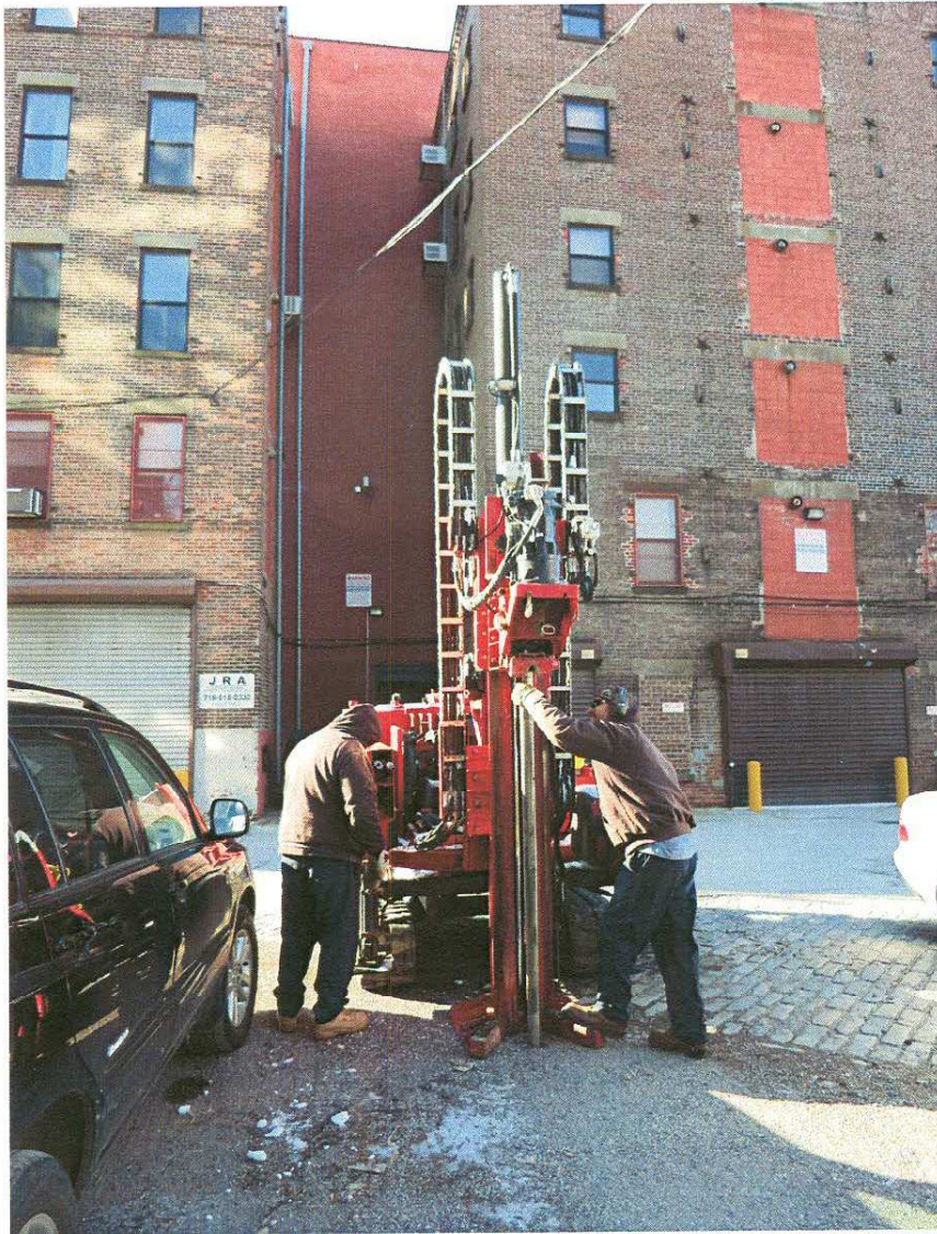
View of Soil Boring and the Surface Material
