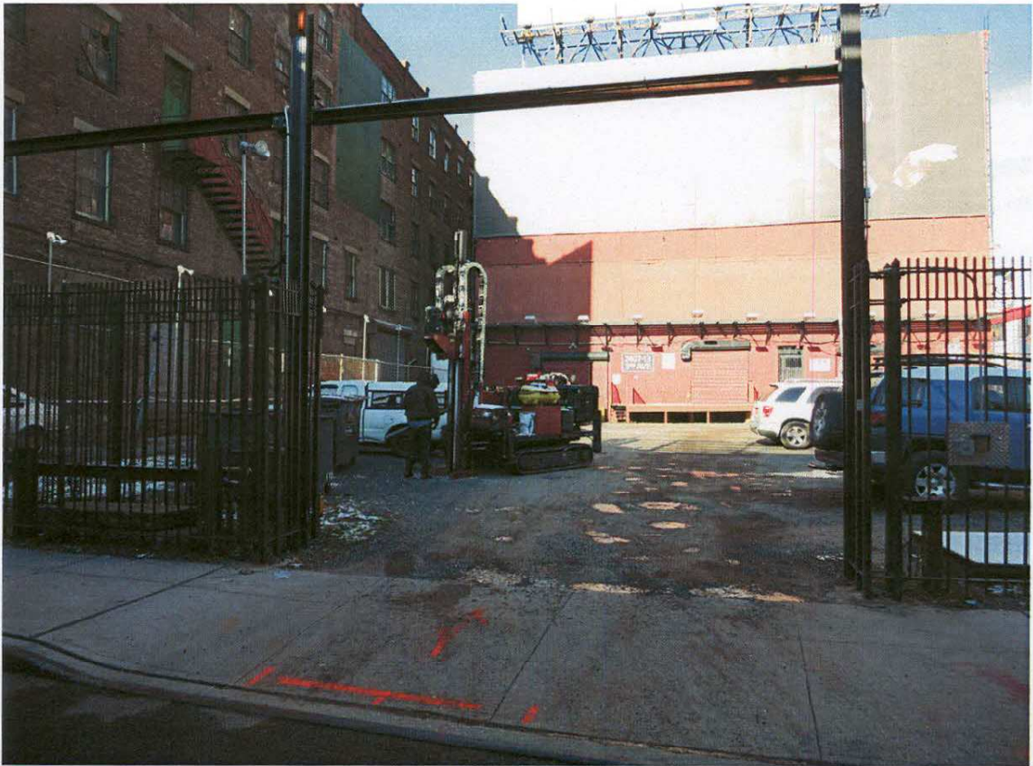
View of the Soil Boring Operation at 2413 3 rd Avenue, Bronx, NY
