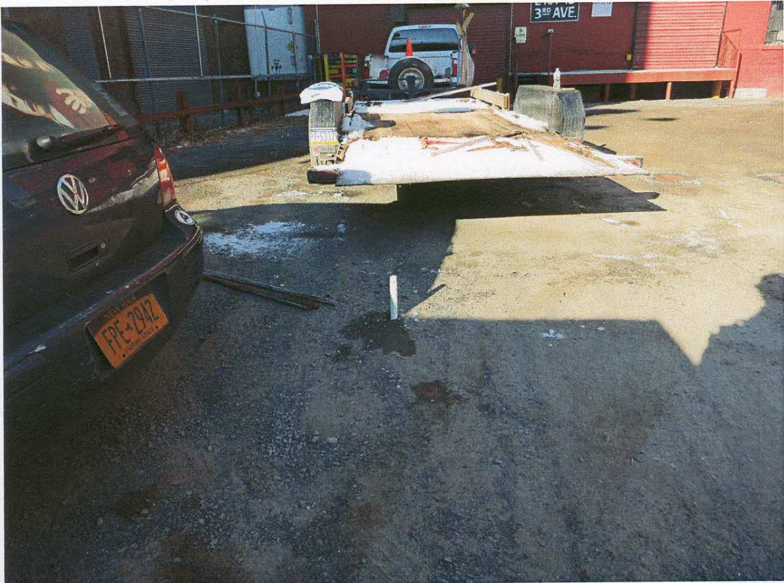
Another View of the Temporary Groundwater Monitoring Well installed at the Location of Soil Boring #2
