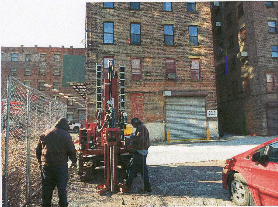
Another View of the Temporary Groundwater Monitoring Well installed at the Location of Soil Boring #2
