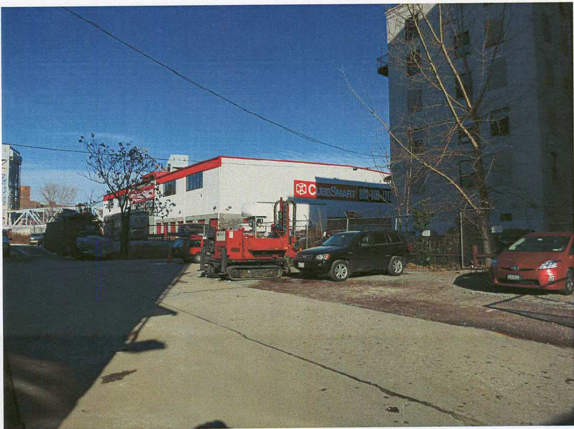
Another View of the Soil Boring Operation
