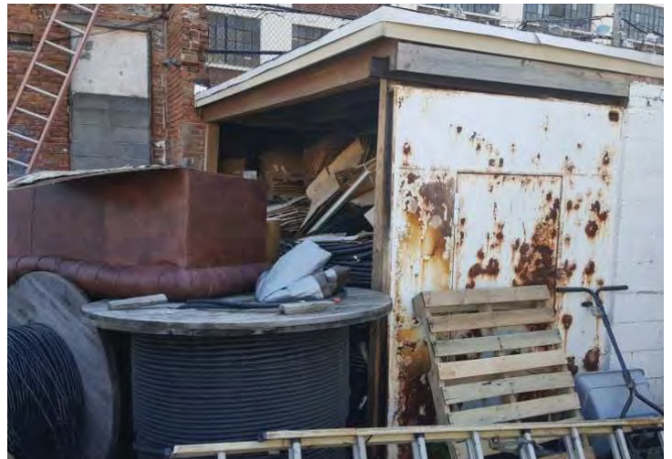
750 E. 134th St. STORAGE SHED
