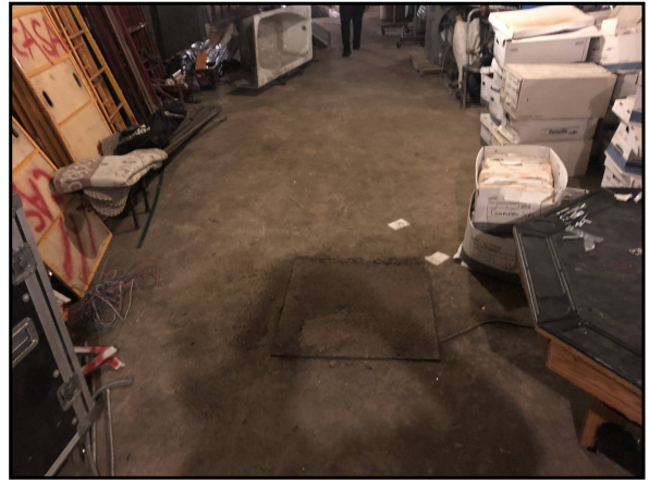
8 : Sump pit in the basement.
