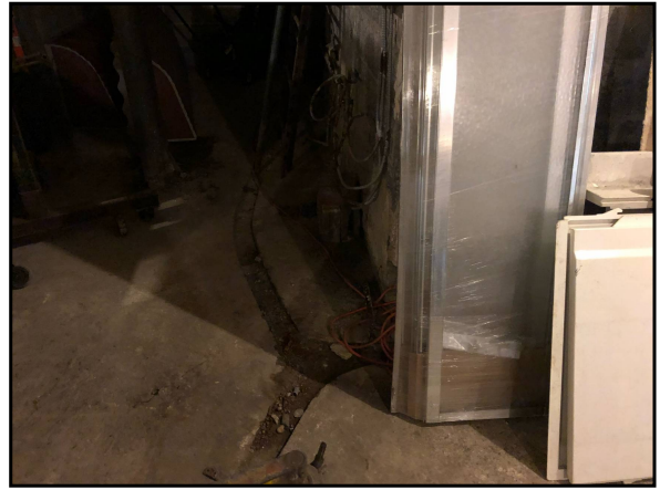
2 : View of trenching with exposed soils on basement floor.
