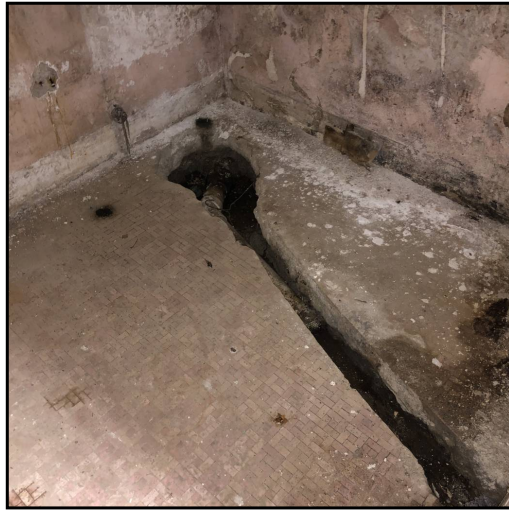
7 : View of trench in basement floor.
