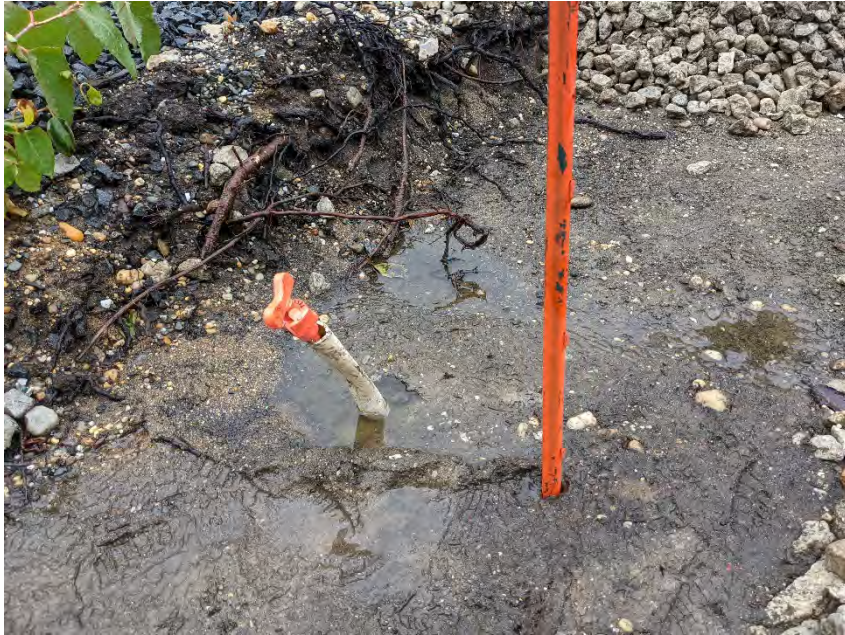
Photograph 15: View of the casing of MW2, which was pinched at the base. This damage prevented the well from being sampled or gauged.
