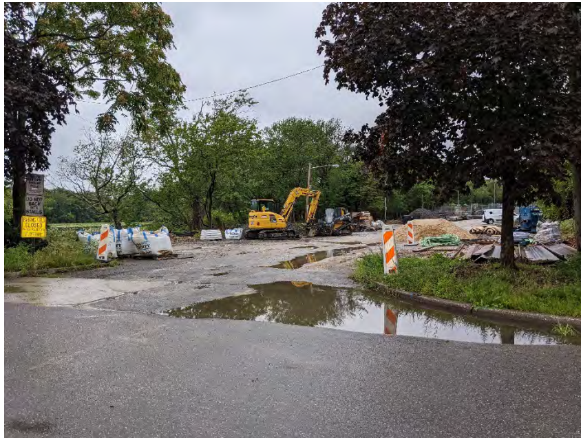
Photograph 1: View of the Site, facing northeast.
