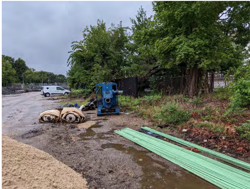
Photograph 3: View of the eastern side of the southern portion of the Site, where MW12 is located.
